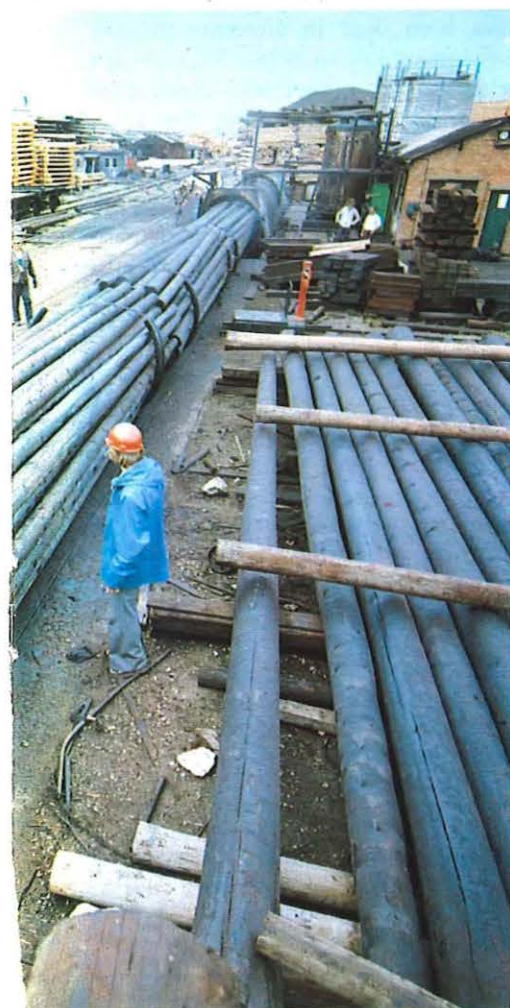
... a creosoting chamber which can
