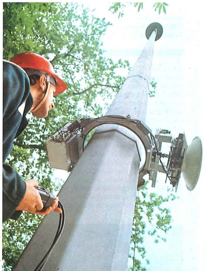
An aerial is raised to the top of an experimental microwave radio mast near Martlesham. The equipment is used in tests of radio-relay systems that will have a greater capacity for carrying telephone calls and television pictures.
