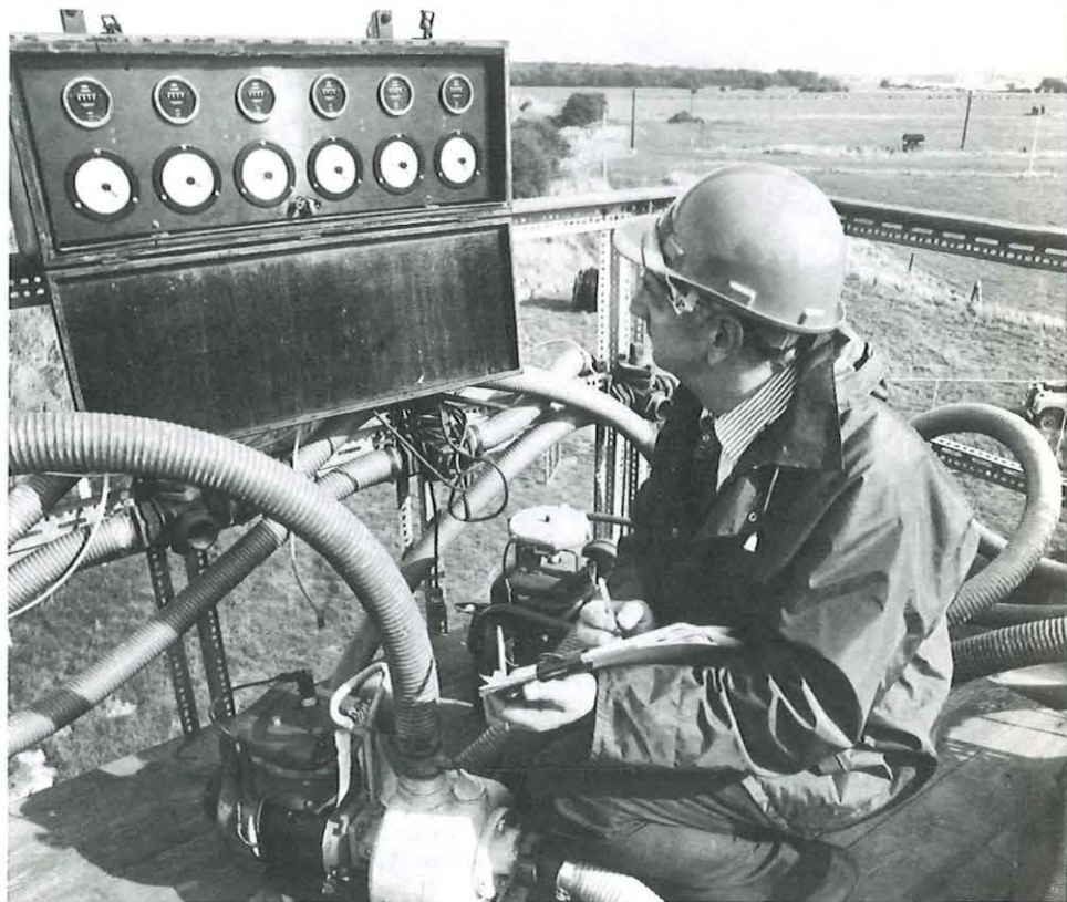
Pumps under test draw water up to the top of this specially erected tower. Performance is measured on a meter panel linked to the pumps.
