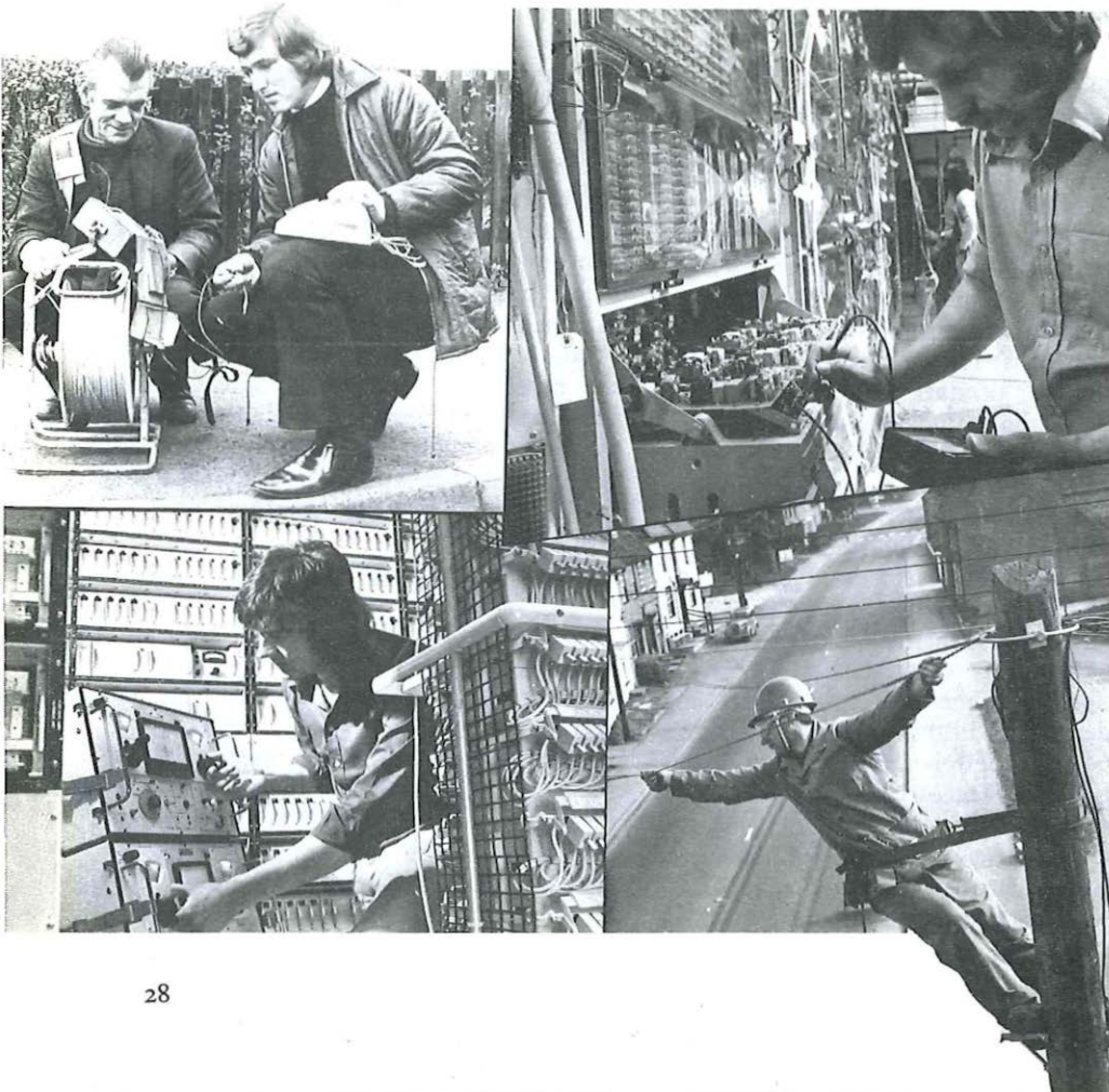
Post Office engineering technicians at work on some of the many tasks they carry out in helping to provide and maintain telecommunications services.
