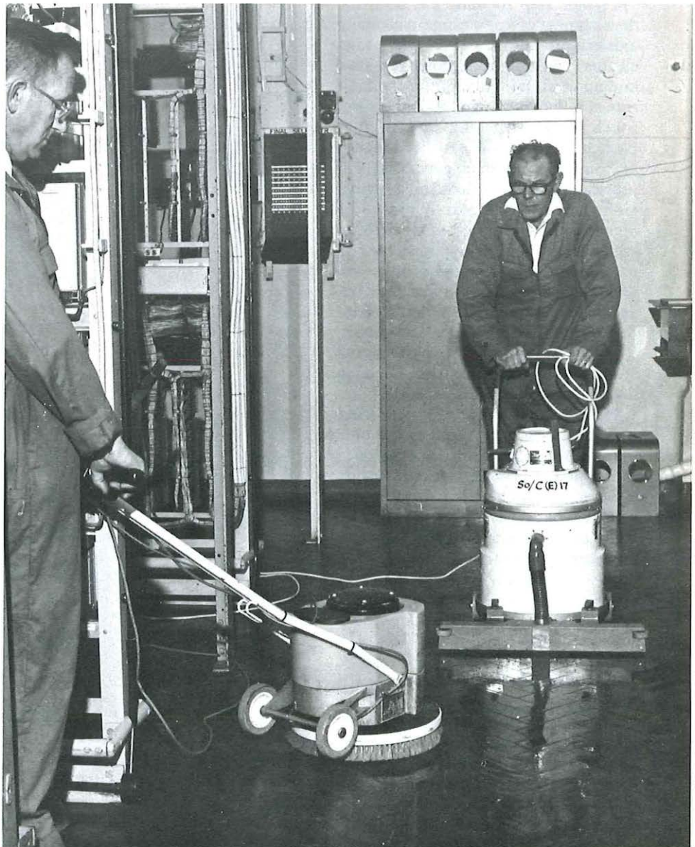
Following removal of old wax from the floor by the scrubbing equipment (left), the area is immediately dried by using a "wet" pick-up machine.
