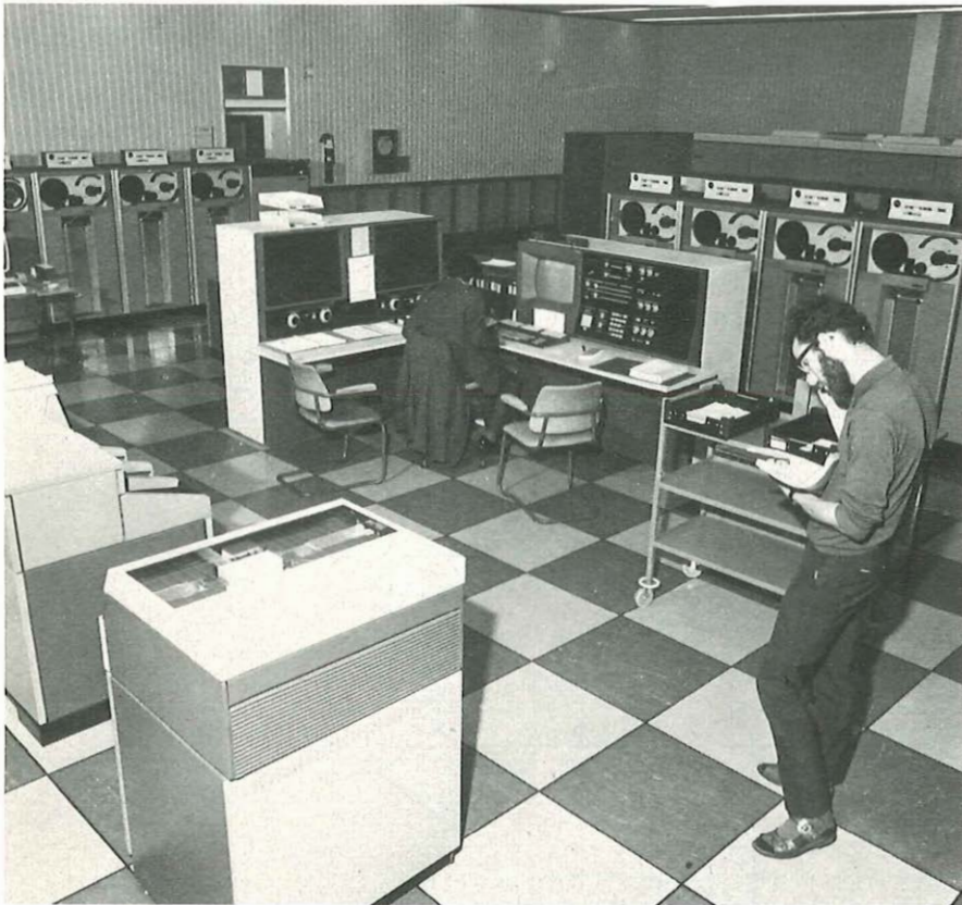
A general view of the Post Office's new IBM 370/168 computer installation at Harmondsworth, which is being extensively used for exchange simulation studies. The control console is shown opposite.
