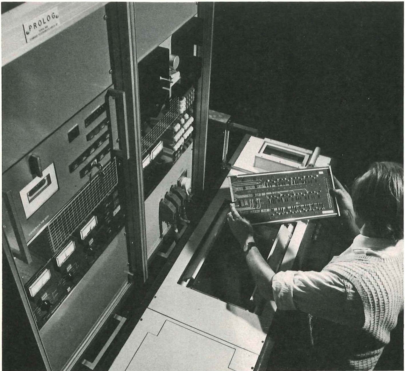
A plug-in electronics unit for TXE4 is checked by automatic equipment designed for production line testing.
