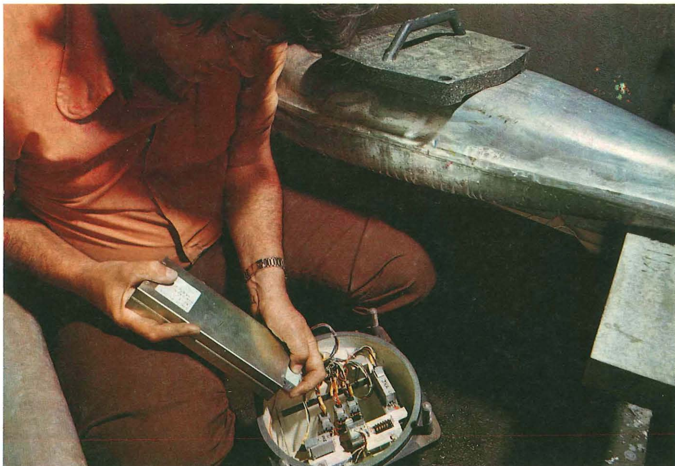
An installation engineer tests a 30-channel pulse code modulation regenerator unit.
