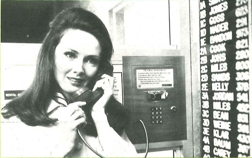
A visitor calls one of the residents in a block of flats by using a push-button telephone unit in the lobby. The residents can unlock the main entrance by dialling a certain number on the telephones in their flats.
