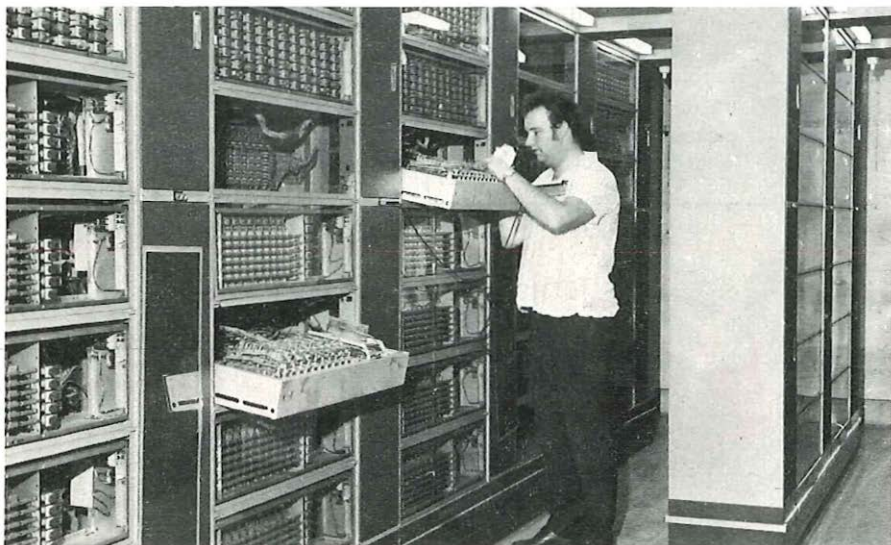
Below: Robin Hughes, Post Office maintenance officer for the telephone system, tests part of the crossbar exchange equipment.
