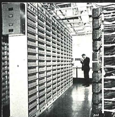
Telegraph Multiplex in London International Telex Exchange.
