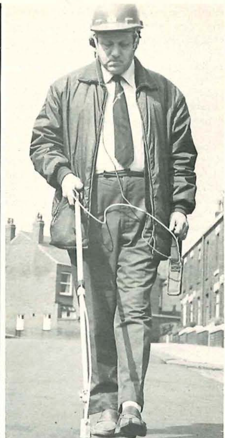
A Plant Protection Officer uses cable locating equipment to find the route of an underground telephone cable. See the item "Protection squad".
