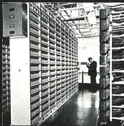
Telegraph Multiplex in London International Telex Exchange.
