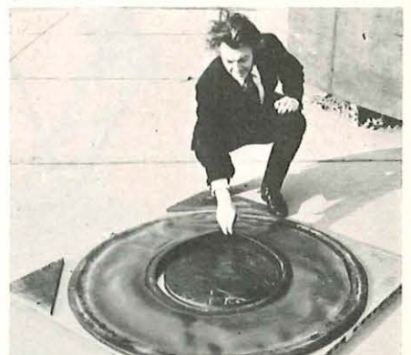
The underside of a platform, showing its flexible bag. Four platforms will be used to move a cable pan, which may weigh up to 80 tons when fully loaded.
