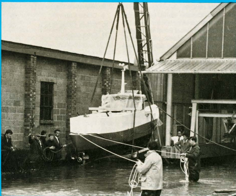
The 1/12th scale model, 24 ft long, goes into the water for the first time in the British Hovercraft test tank at Cowes, Isle of Wight.
