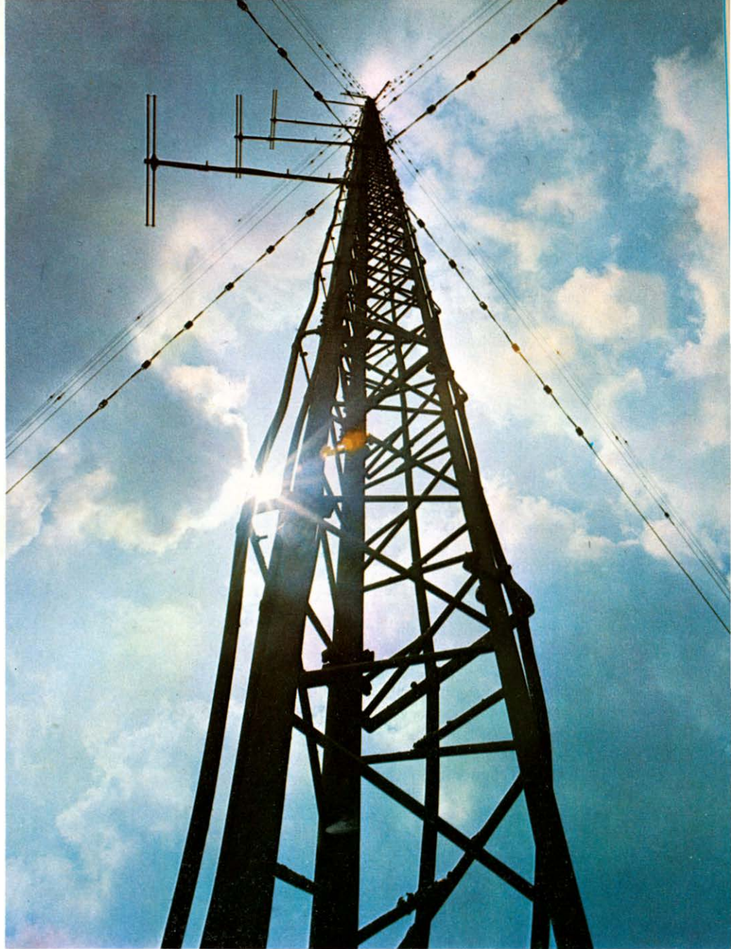
The mast at North Foreland Radio Station.
