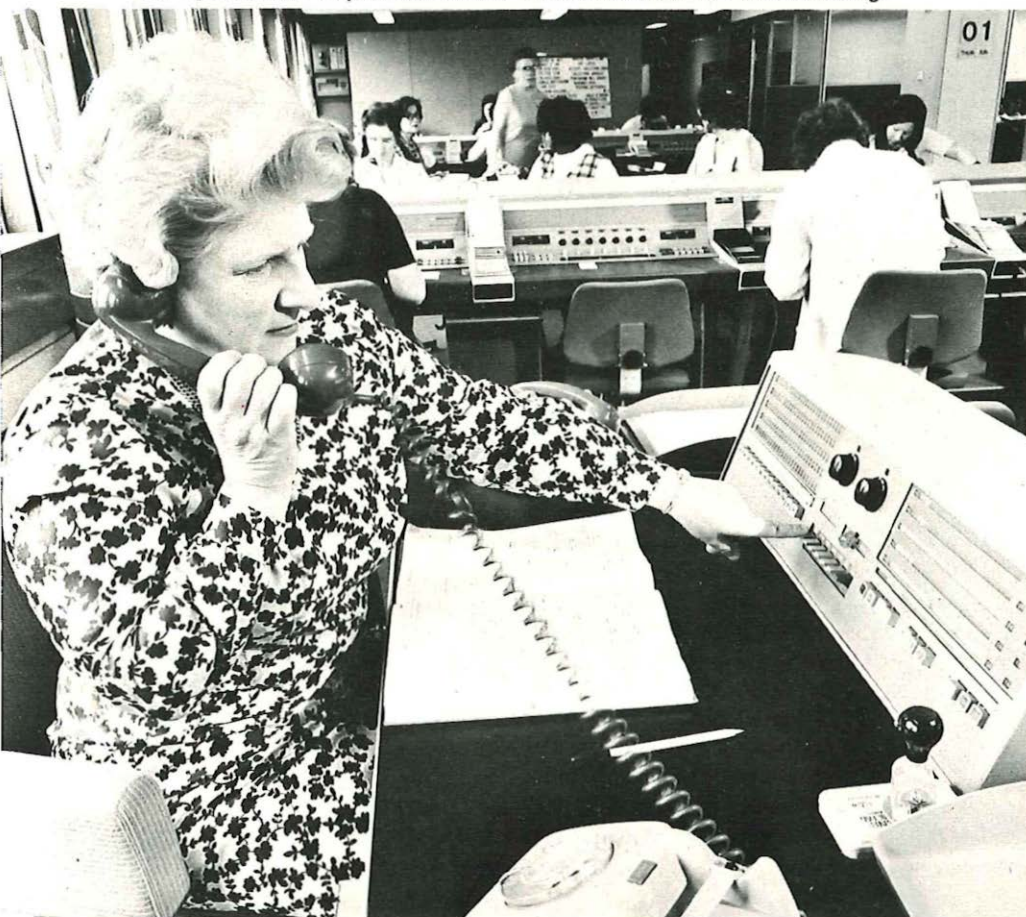
An Operational Supervisor at her control console in Fleet Building.
