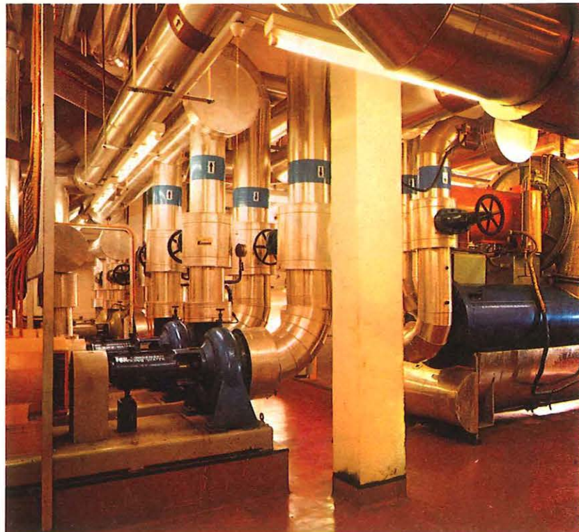
Part of the refrigeration machine plant which supplies cold water to the air-conditioning system. It cools the air in all apparatus space and switchrooms.
