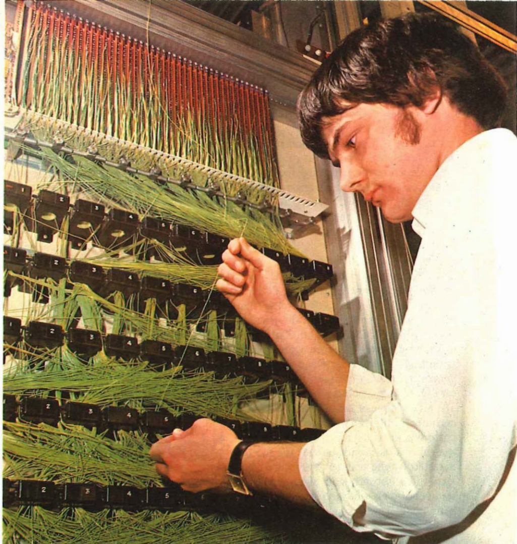
Threading a subscriber's wire in the cyclic-store area.
