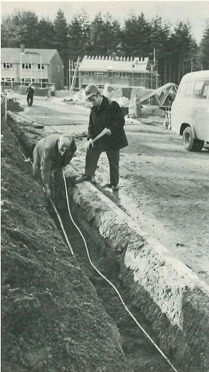
Left: Telephone and electricity cables are laid side by side during a "twinning" job at Bracknell, Berks. The Housing Estates Liaison Officer for Bedford Telephone Area discusses the job with the foreman of the Electricity Board gang which laid both cables.
