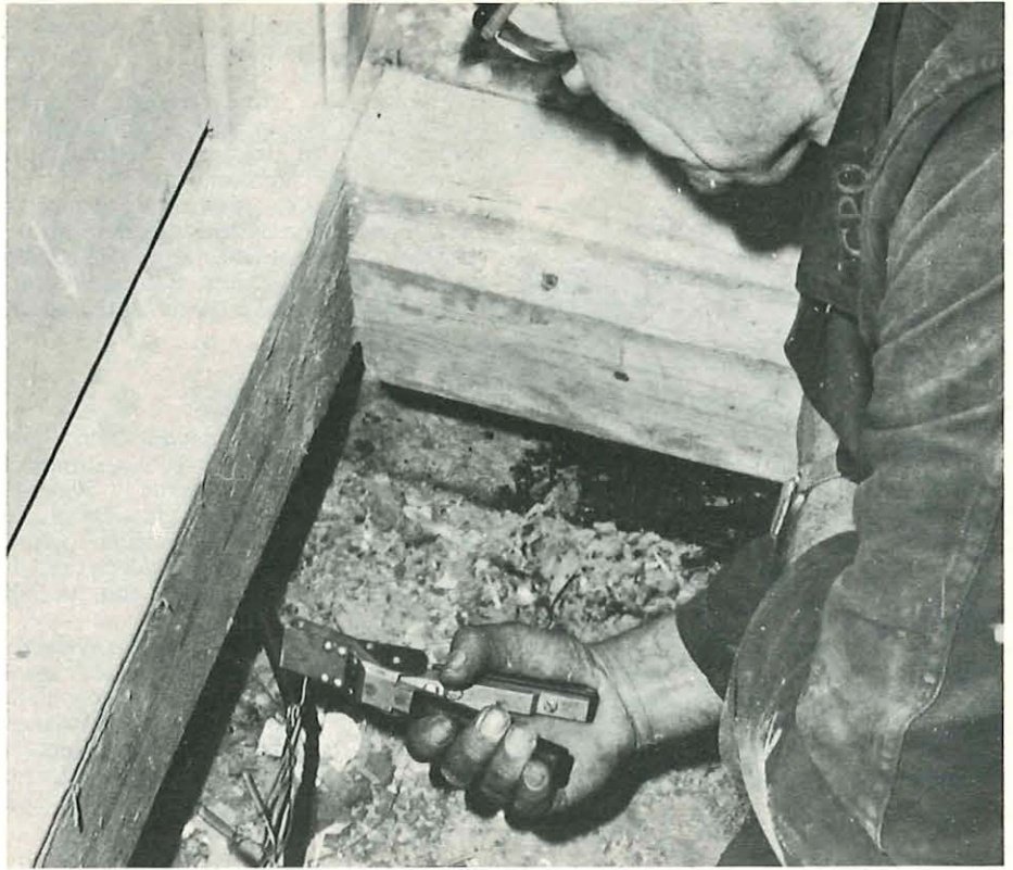
Making a joint in the cable at one of the Aboyne houses. The jointer has quick and easy access to the cable from the trapdoor.
