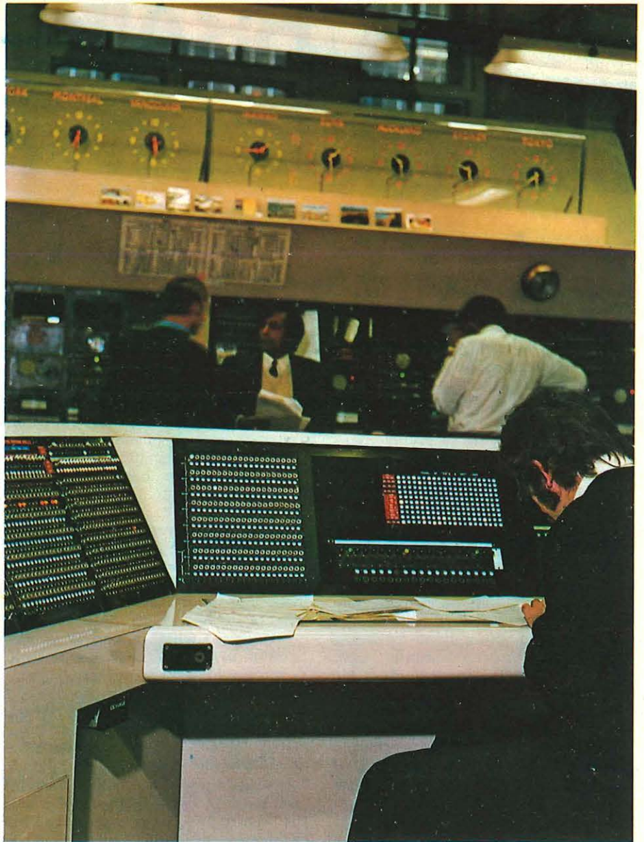
Above: Dave Locke, an Assistant Executive Engineer, examines the miniature relays which are reducing call-queueing problems. These little electronic devices "sense" a build-up of waiting calls and switch them to a free route much more quickly than before.
