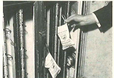
The old Desiccator with solid casing and (right) the new type—a throw-away bag.
