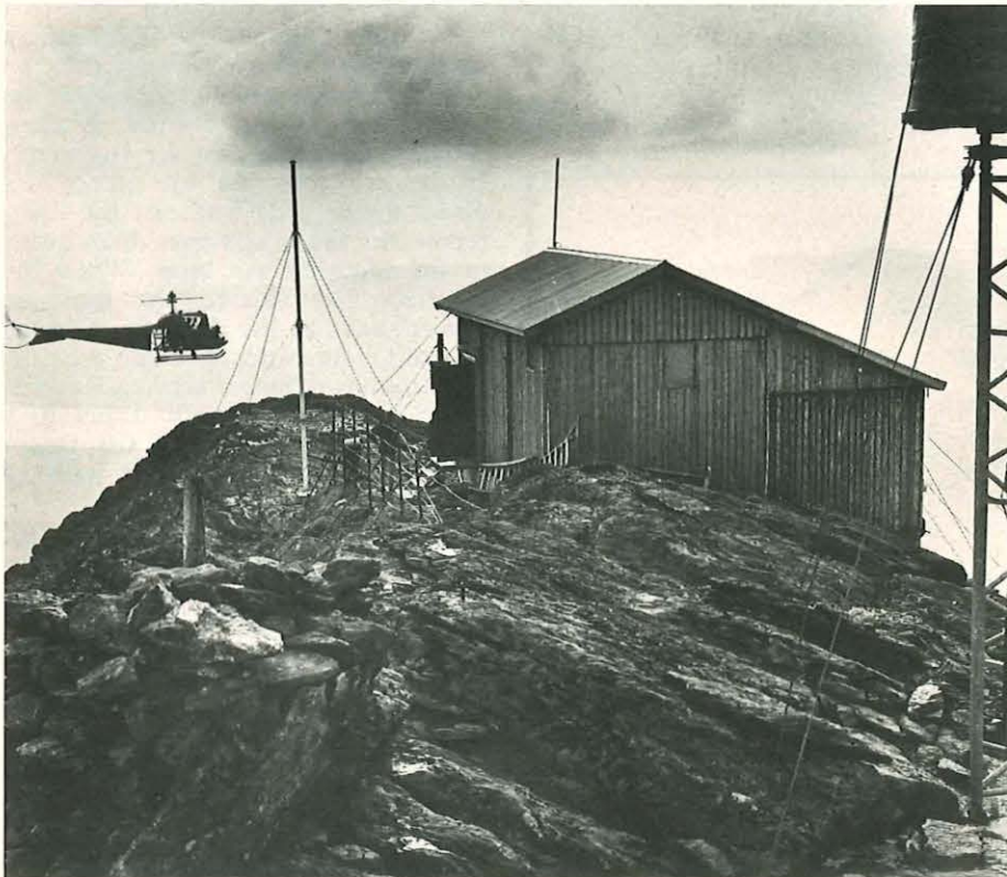
A helicopter flies in material for the construction of a microwave radio tower in the mountains of North Sweden.
