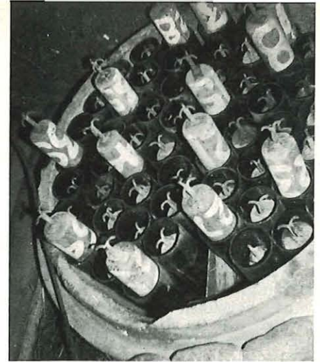
Left: Laying ducts in the 36 in-diameter pipe, made of thick concrete, which is thrust through the soil in sections.
