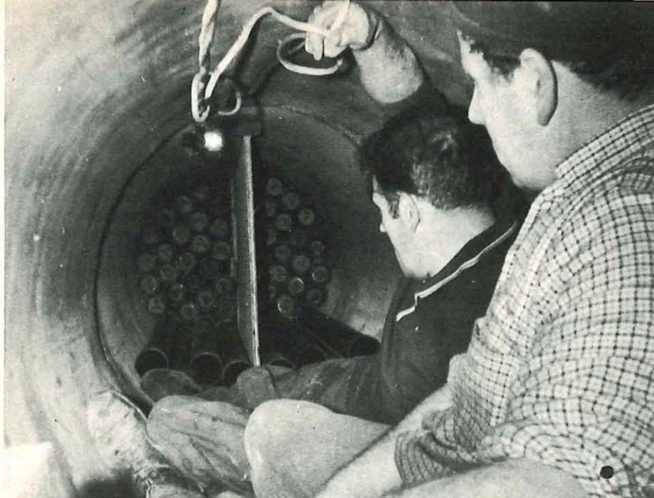
Left: Laying ducts in the 36 in-diameter pipe, made of thick concrete, which is thrust through the soil in sections.
