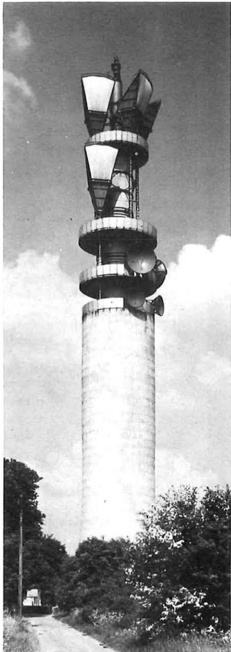
LEFT: The ferro-concrete tower at Wotton-under-Edge. There are several of this type in the network and their shape is well suited to carrying horn aerials though dishes can also be fitted. A limitation of the taller towers of this type is a need to cluster all the aerials at the top which results in excessive aerial height and waveguide attenuation for some directions of shoot.
