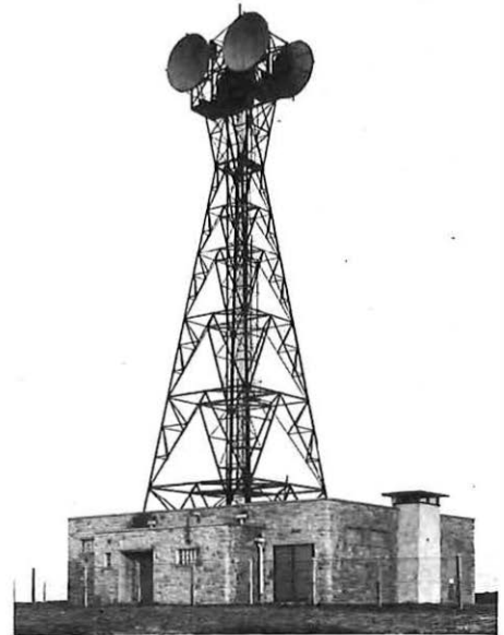
BELOW: Windy Hill Relay Station, which is on the 4 GHz system, was installed in 1952 between Manchester and Kirk o' Shotts primarily to extend television service to Scotland. This route, now recovered, was distinguished by towers of symmetrical and elegant design but their aerial carrying capacity was inadequate to cater for long term growth in the demand for circuits.
