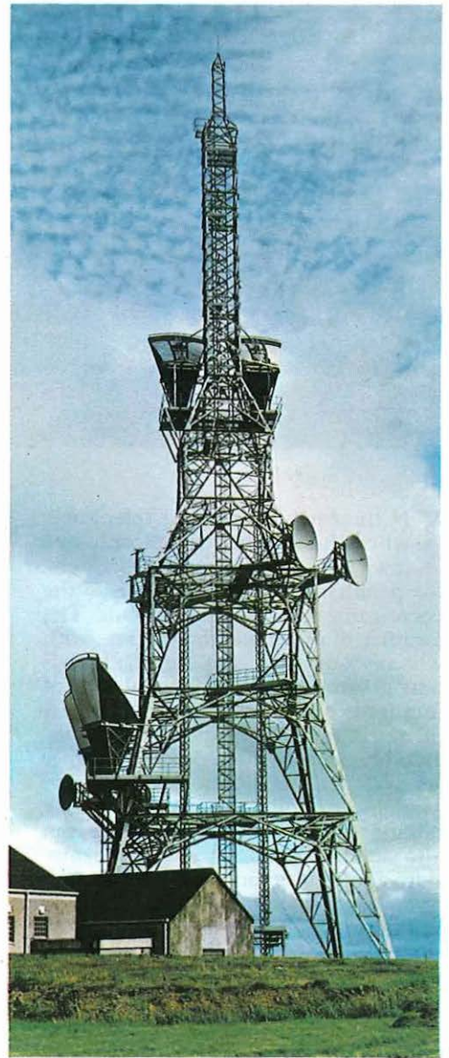
ABOVE, LEFT: This lattice steel tower at Copt Oak Radio Station near Leicester is built in the so-called Eiffel form though its outline is unavoidably marred by the substructures needed to carry the dish and horn aerials. Forecast traffic growth indicates that this tower will eventually be inadequate and its replacement will provide an opportunity to replace it with a tower of more pleasing shape.
