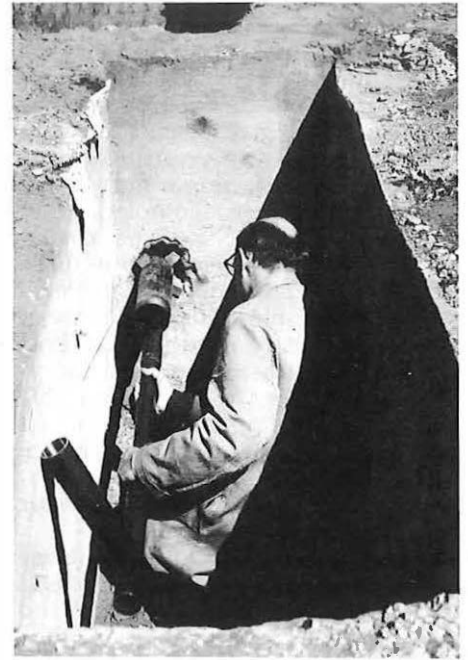
An experimental length of waveguide is inserted into an underground duct.
