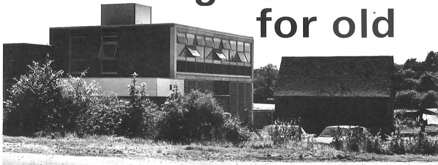
At Highclere, near Newbury, a new TXE2 electronic exchange (left) stands beside the small UAX13 exchange building. The electronic equipment will shortly replace the 25-year-old UAX13.
