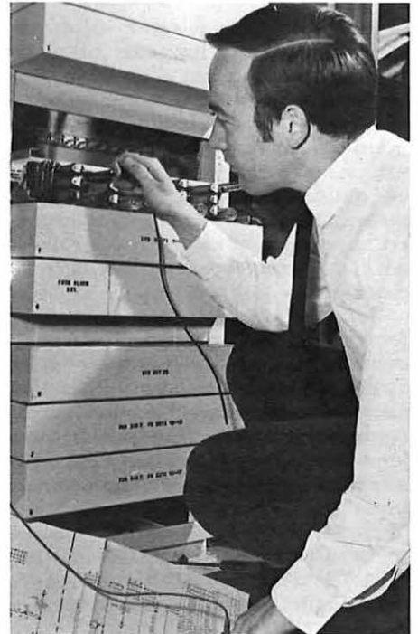
A technician tests the switchboard at the Enfield factory.
