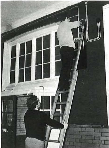
Wiring a school in Bermondsey.
