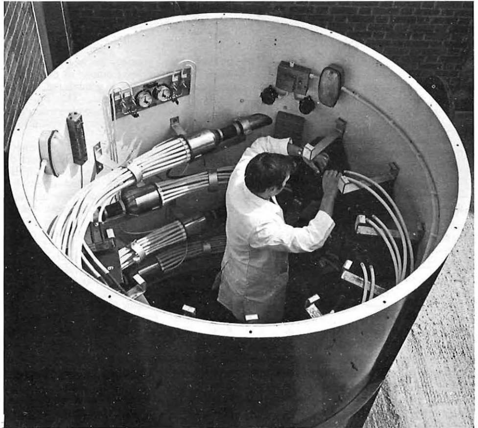
This cylindrical tank will be used in a field trial as a manhole to house the repeaters for the new cable system. Based on the concept of the agricultural silo, it is constructed of steel plate, is 1.8 m. in diameter, 2.4 m. deep and can be sunk in the ground. The coaxial pairs are laid out around the circumference, each being connected to its individual repeater case on the wall. The cable leaves the silo on the same tangent as it enters avoiding sharp bends. The cables are plumbed into entry seals to ensure the installation is watertight.
