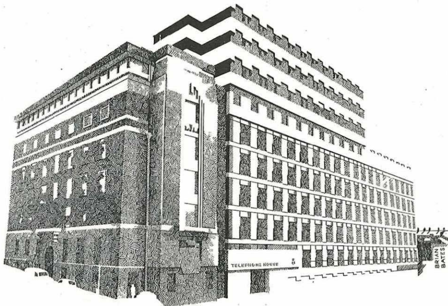
An artist's impression of Telephone House, Birmingham, showing how the old and the new buildings are joined. On the left is part of the old block with an extra storey built on top. On the right is the new section, including the tower block.
