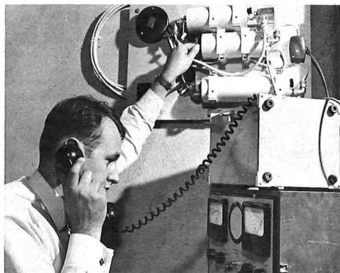
Receiving equipment is commissioned in an office building.
