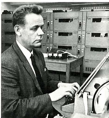
An operator makes a test call through the ITAT equipment. In the background the banks of auto-ticketing equipment which record the calls.
