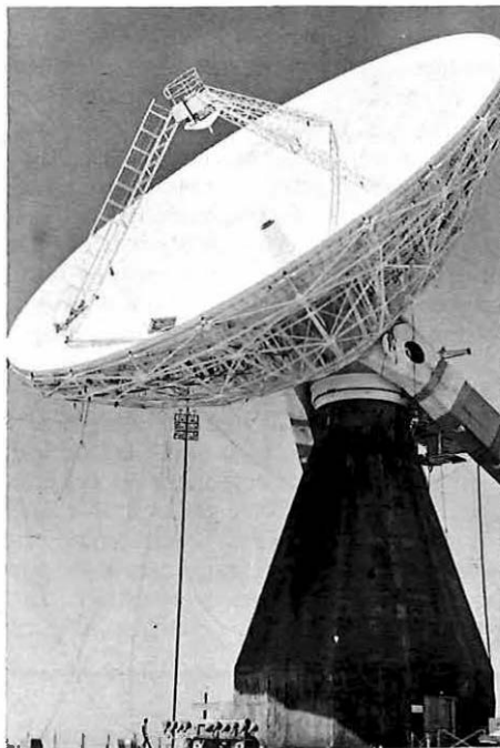
The Earth Station aerial at Bahrain
