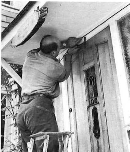
An engineer fitting a lead into a customer's house.
