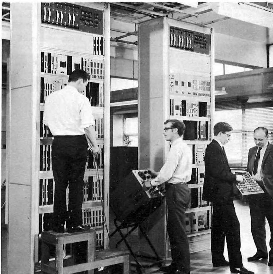
Engineers check a pulse distribution amplifier and monitor circuits in the pulse code modulation equipment at London's Empress Exchange.
