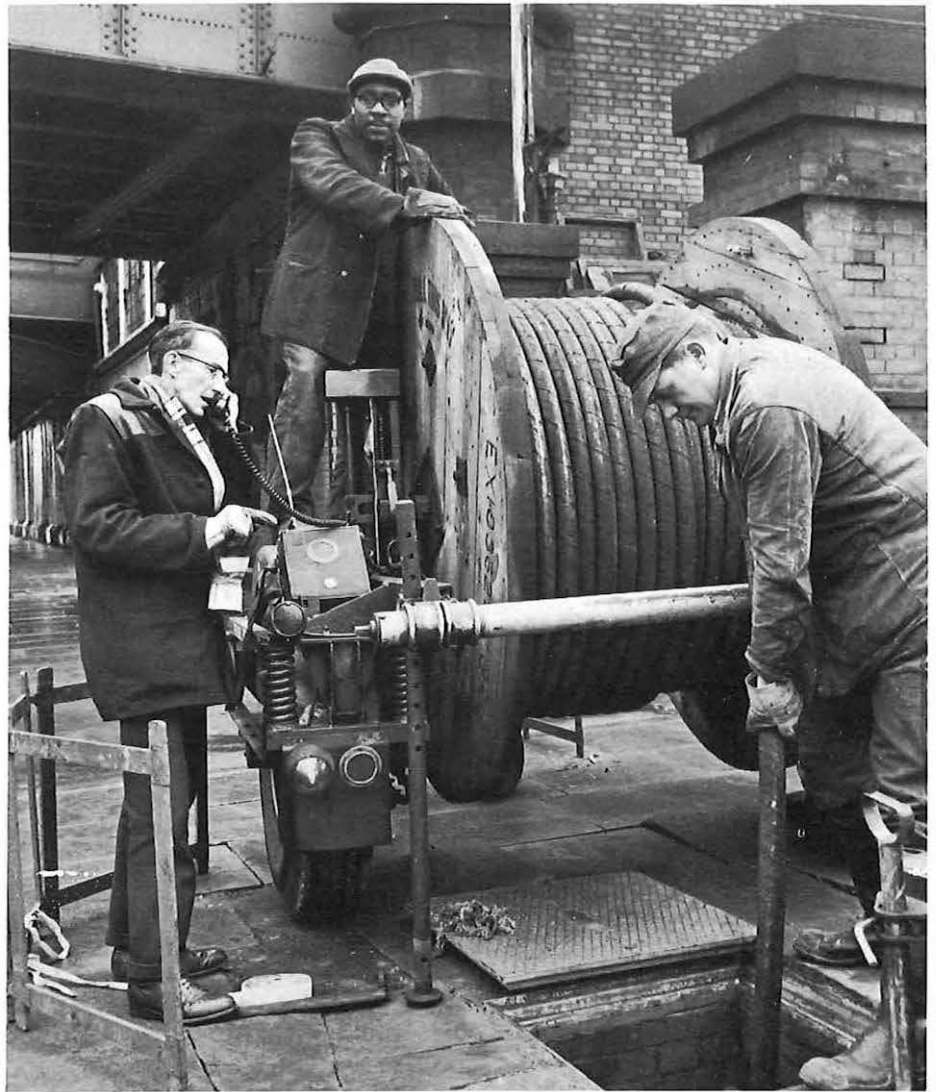
Engineers feed in a main underground cable.
