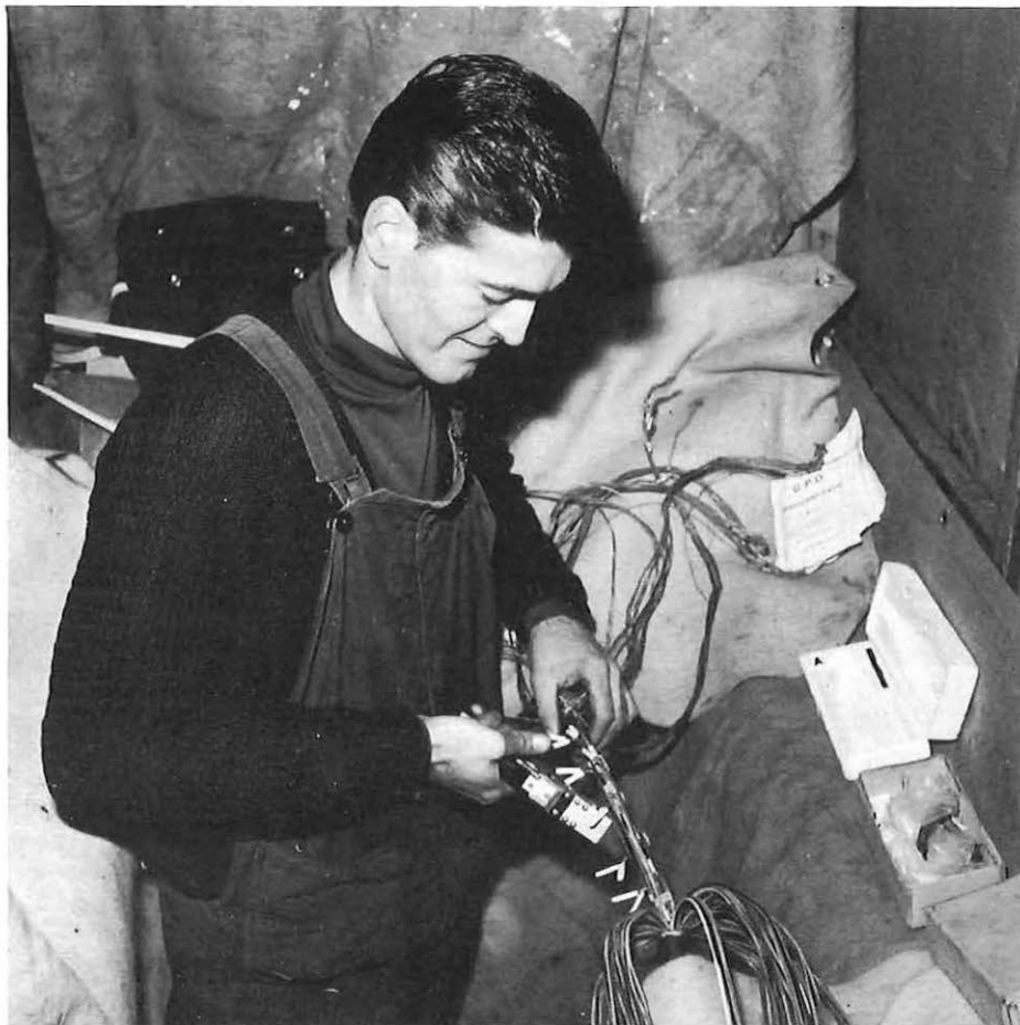
Mr. R. A. Hoare a Tech 2A using "B" wire connectors and crimping tool.
