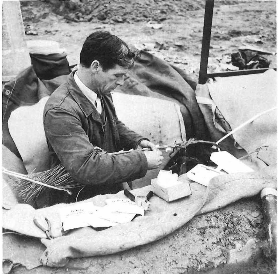
Tech 1 Mr. S. R. Hoverd jointing the aluminium cable to a copper tail.
