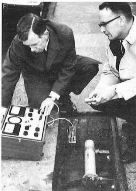
Mr. N. J. Tolcher checks the signal level at a joint box repeater while Mr. K. J. Trussler looks on.
