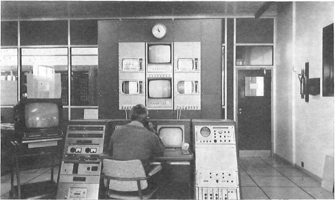
A general view of the colour television monitoring console at the Goonhilly satellite earth station.
