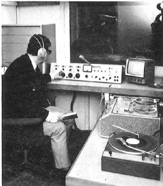
The sound control room at Leeds is equipped with a record player, tape recorder, monitor screen and control console.
