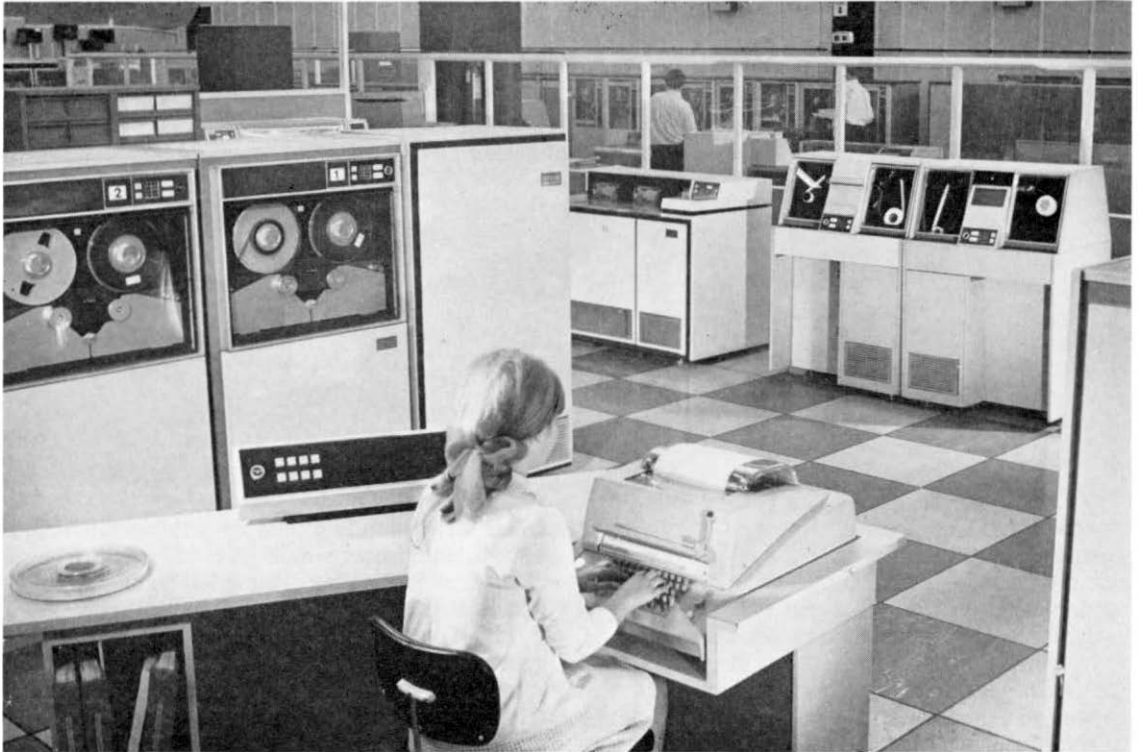
A general view of the equipment now being installed at Bootle, being tested at the manufacturer's works.
