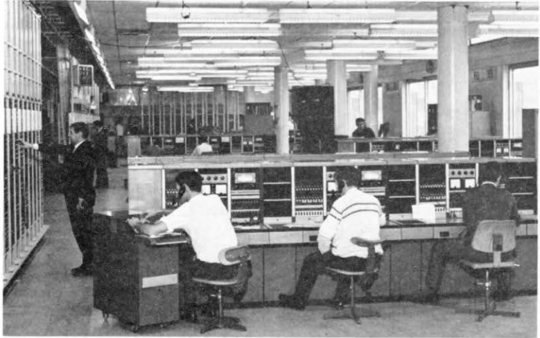
The Test Room—focal point of the building—showing the suite of test jack frames and some of the test desks.
