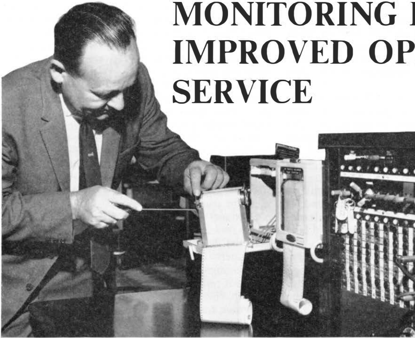
An engineer makes adjustments to one of the new monitoring devices at Palmers Green exchange.
