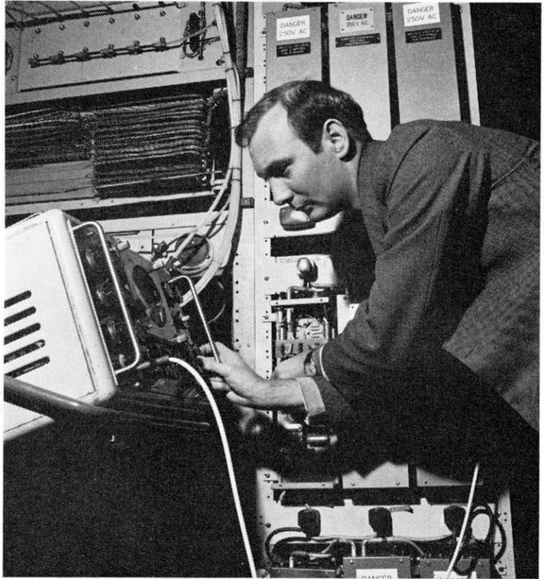
Technical Officer A. Stone adjusts the video amplifiers at the Belgravia Telephone Exchange.
