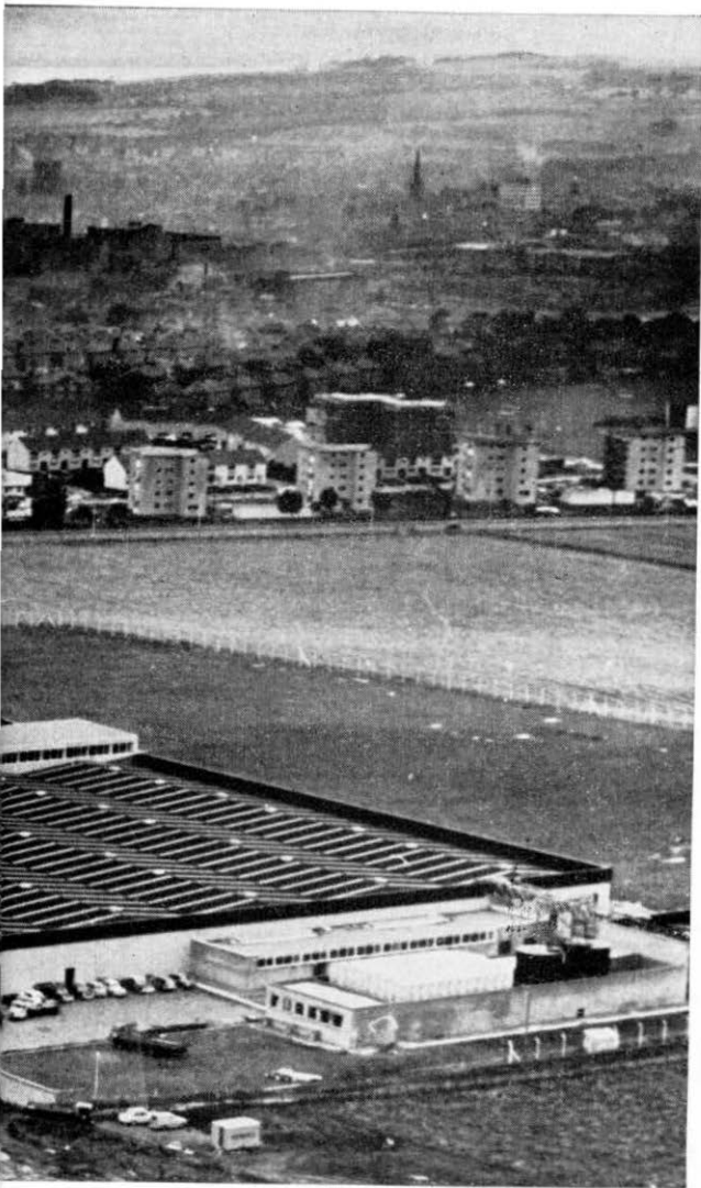
The new 258,000 sq. ft. AEI telephone exchange equipment factory at Kirkcaldy, in Fife
