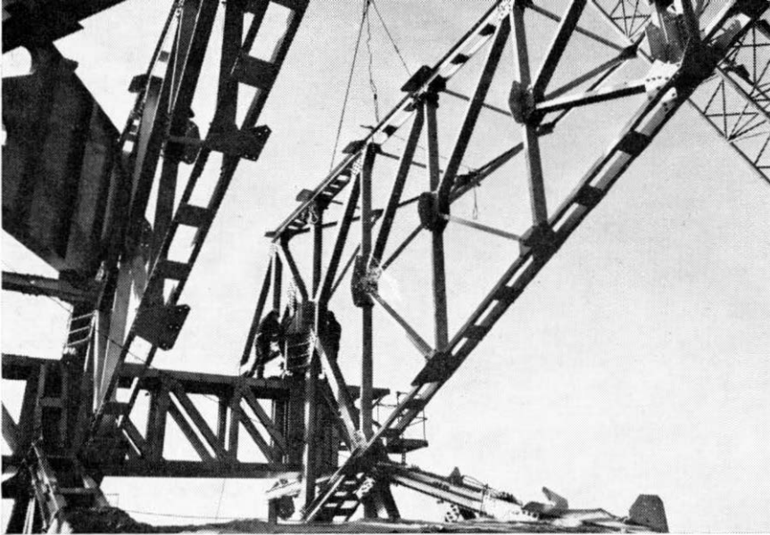
An assembly gang prepares part of the reflector backing structure for the new aerial.
