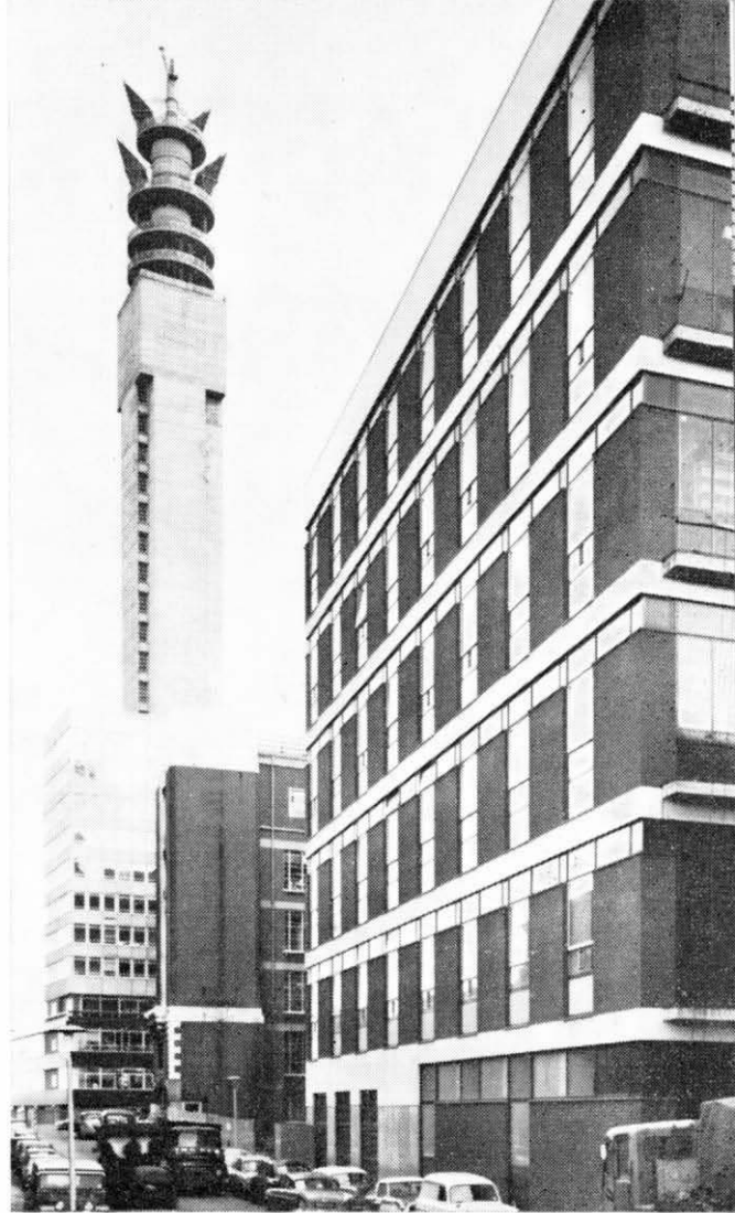
Part of the recently-completed extension to Telephone House, Birmingham. In the background is the new Post Office Tower, one of a network of microwave relay stations which the Post Office is setting up throughout the country.
