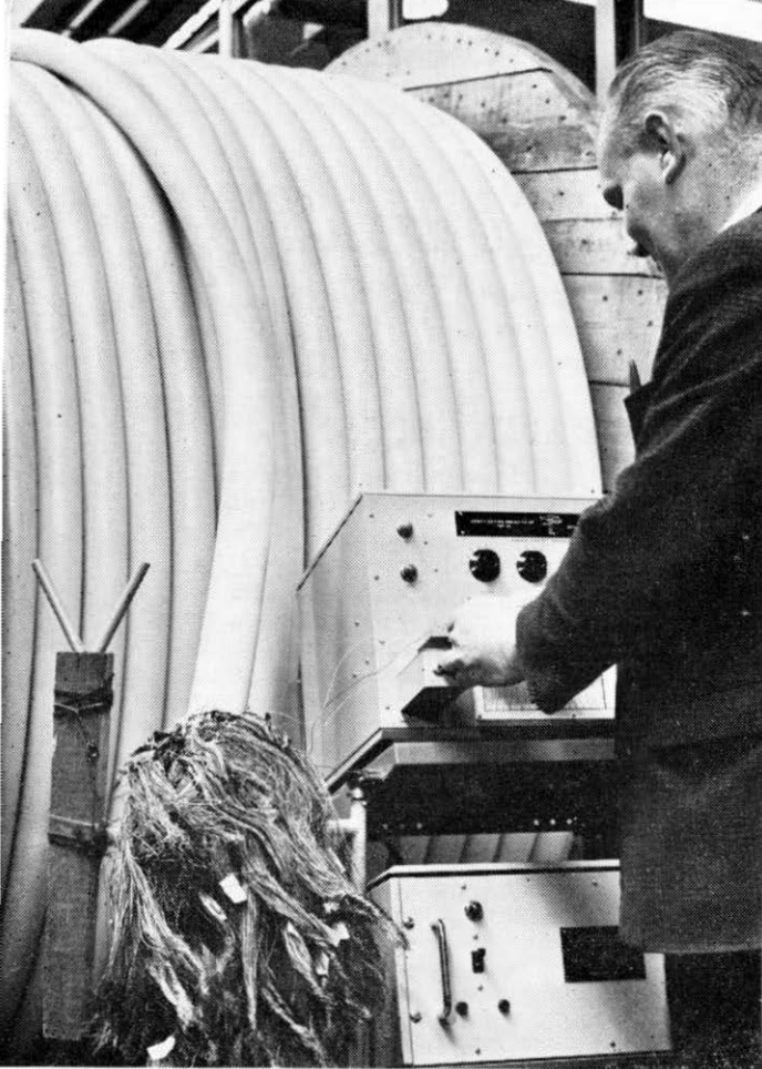
An engineer testing the new telephone cable which contains more pairs than ever before, accommodated in a single cable suitable for installing in a GPO standard duct.
