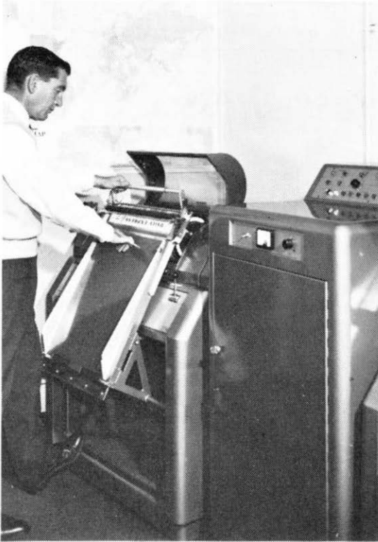
Above: A Daily Express picture telegraphist loads a page proof on to the drum of the transmitter. Right (top): Less than 20 minutes later in the offices of El Mundo, a photo-sensitive film is made of the front page and (bottom) two model girls in San Juan read the very latest news from London.
