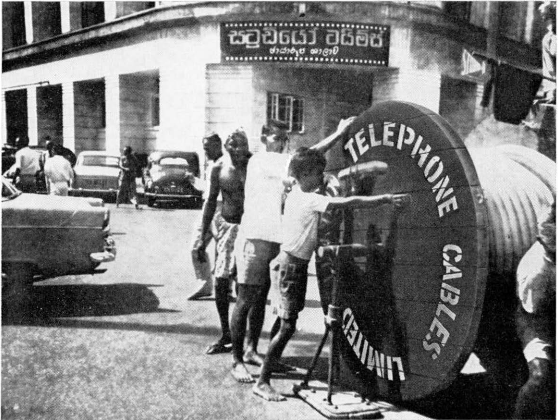
TCL cables being laid in Main Street, Colombo, Ceylon
