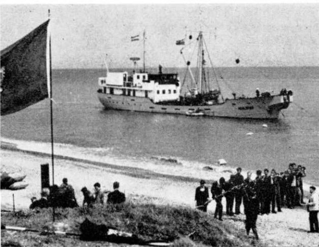
The shore-end cable is hauled ashore from the Dutch cable ship Poolster as she lies off Coverhithe. The new cable will have a capacity of up to 480 circuits.
