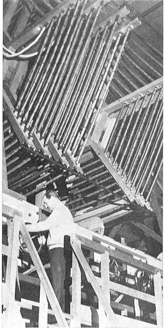
Above (left): A Technical Officer checks the connections to one of the three final stage, vapour-cooled valves. Right: Technical Officer Mr. A. E. Christopher adjusts a tapping switch on the aerial tuning inductance coils.
