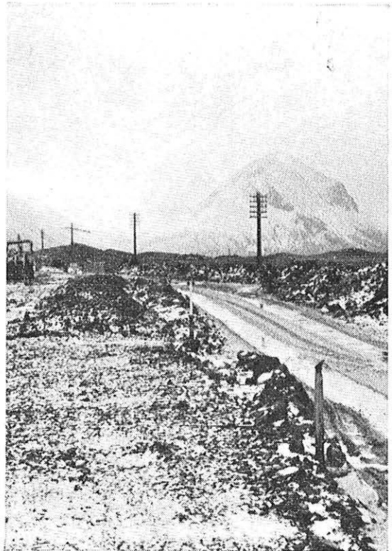
On the road between Inverness and Ullapool between which a new coaxial cable system will be laid to replace the existing open wire route.
