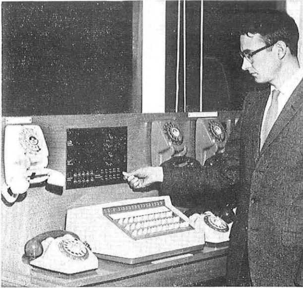
Mr. J. A. Carlisle, a senior engineer of the Plessey Telecommunications Group, operating a display panel at the new Ambergate Exchange. The panel indicates numbers being called.
