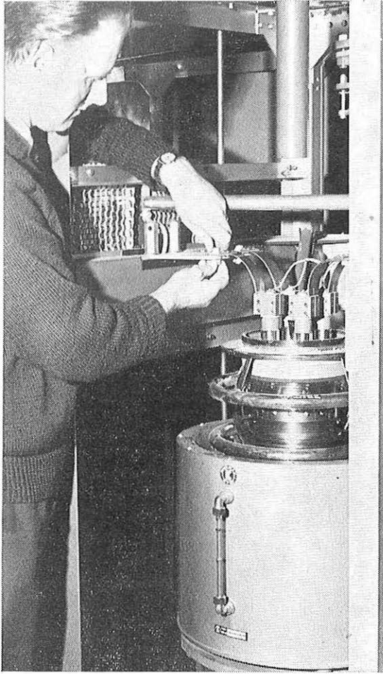
Above (left): A Technical Officer checks the connections to one of the three final stage, vapour-cooled valves. Right: Technical Officer Mr. A. E. Christopher adjusts a tapping switch on the aerial tuning inductance coils.
