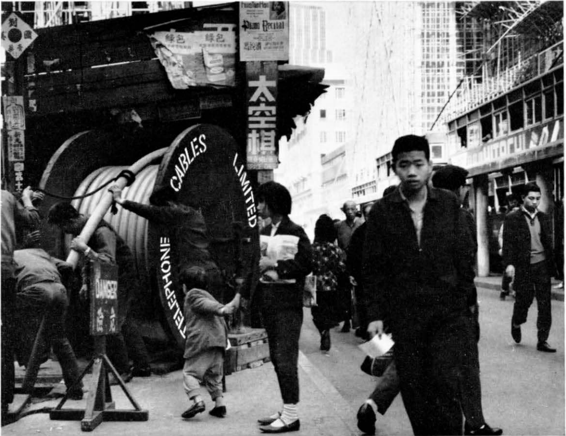
TCL cables being laid in the main business centre of Hong-Kong
