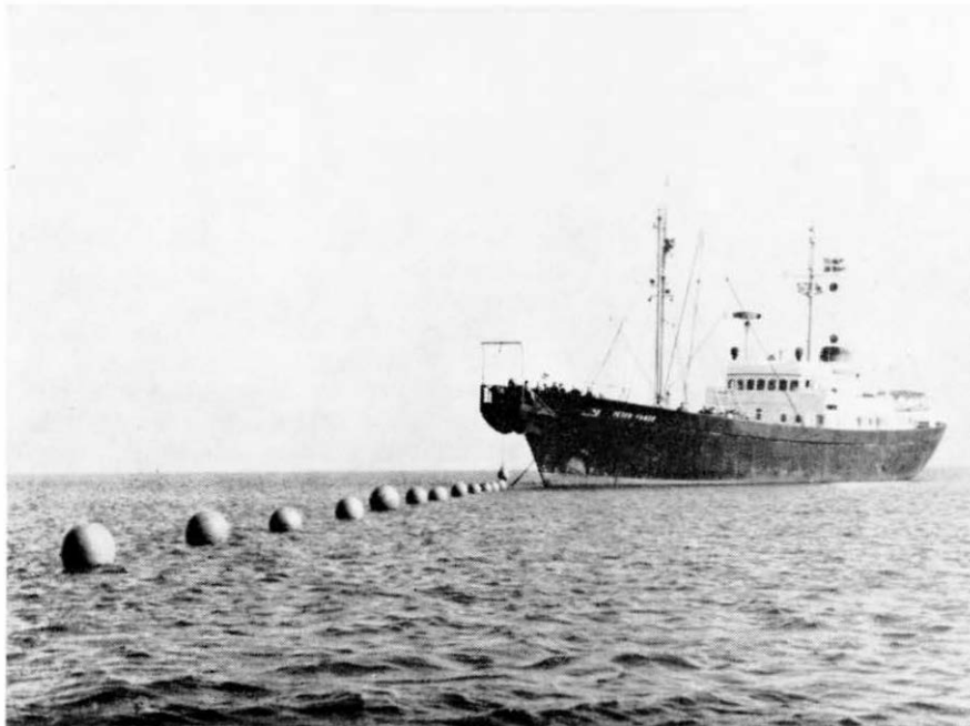
The shore-end cable being laid at Cayton Bay, Scarborough.
