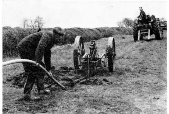
Above: Laying two-inch pipe with the Ransome CIE Moleplough. Below: Tensioning the steel wire which holds lengths of pipe together as they are drawn into the ground.
