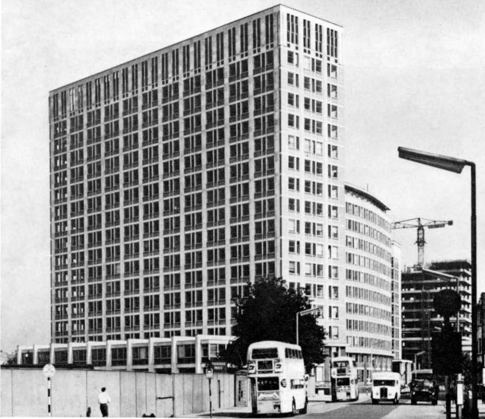
Camelford House, the Headquarters of LTR, towers above the Thames on the Albert Embankment.
