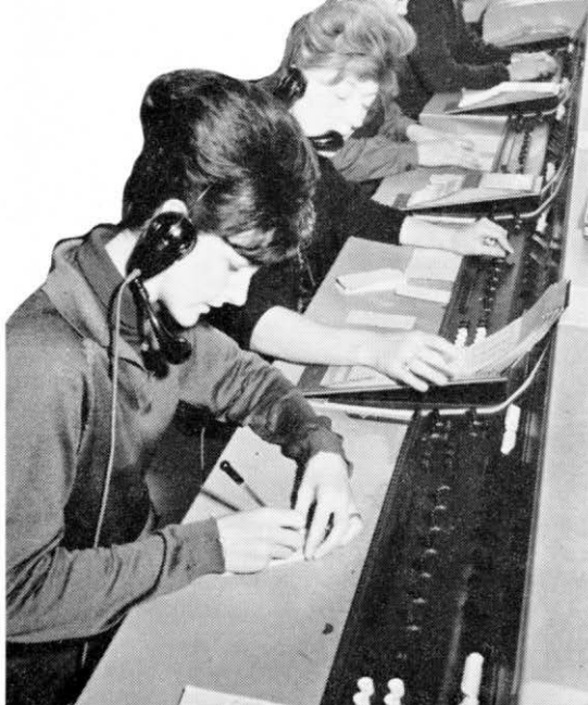
Operators at work on the new cordless switchboard which is being installed in all new exchanges. The new boards are easier to handle and less noisy.
