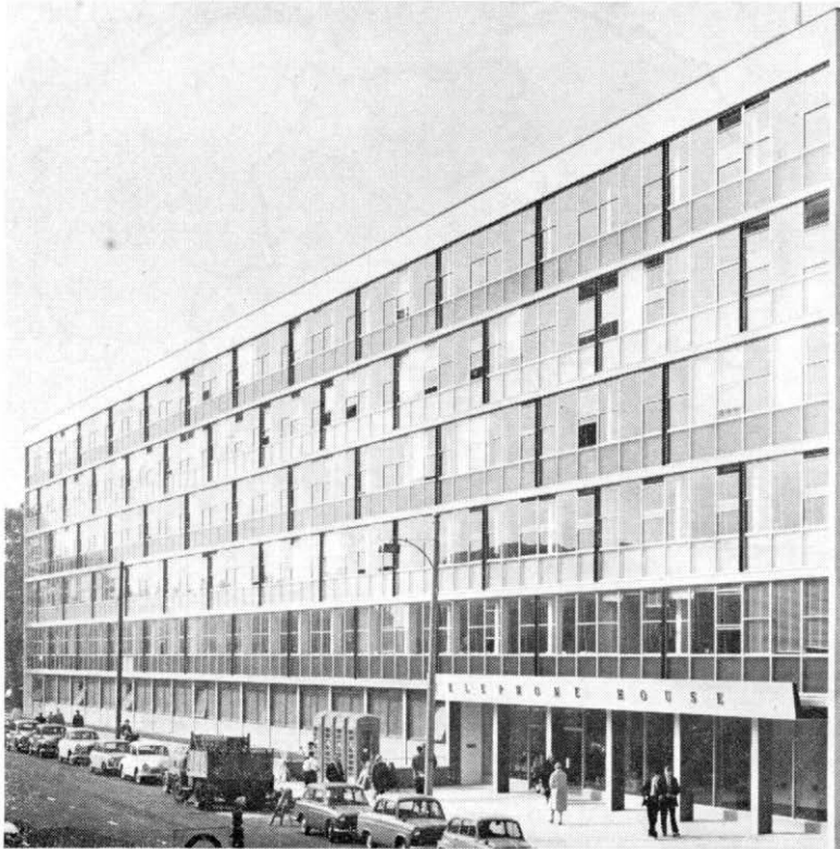
The South-West Area Telephone Manager's Office in Wimbledon, which has been relieved by the setting up of the new South Area.
