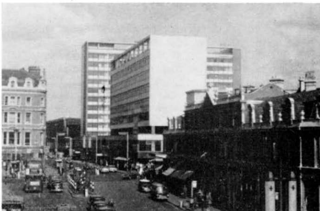
The new relay unit will be installed in Cardinal House, Farringdon Road, the tall building in the background which is partly covered by Caxton House. The unit will be ready for service in 1967.
