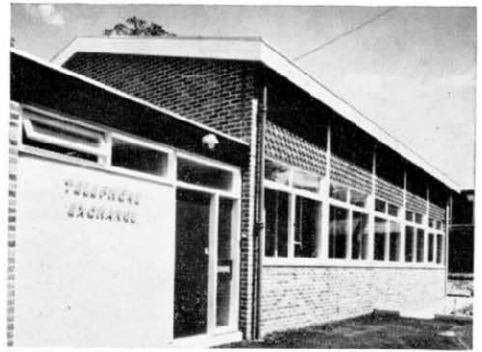
Above(left): Wantage automatic telephone exchange, built in 1964, is an example of the K1, Mark IV design using traditional building methods. Right: The H-type now replaced by the L and K designs.
