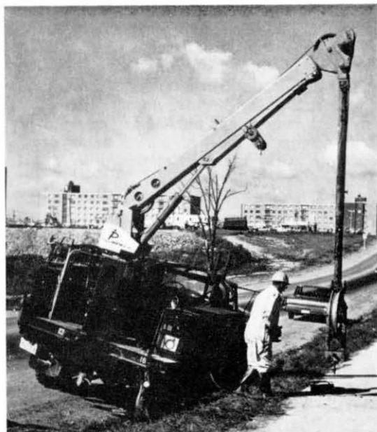
Above: A Canadian construction vehicle which pulls cable through ducts very rapidly. Below: The Pentax electronic exchange recently introduced at Peterborough.
