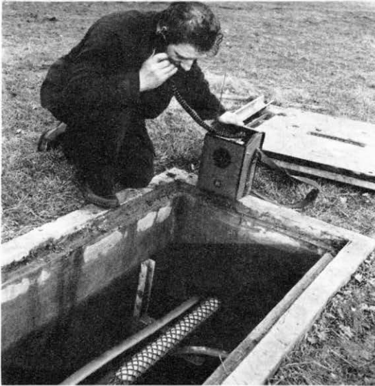
A technician uses a portable radio to report the arrival of a cable at a jointing point. A loudspeaker is incorporated in the set to leave the technician's hands free when it is necessary for him only to listen.
