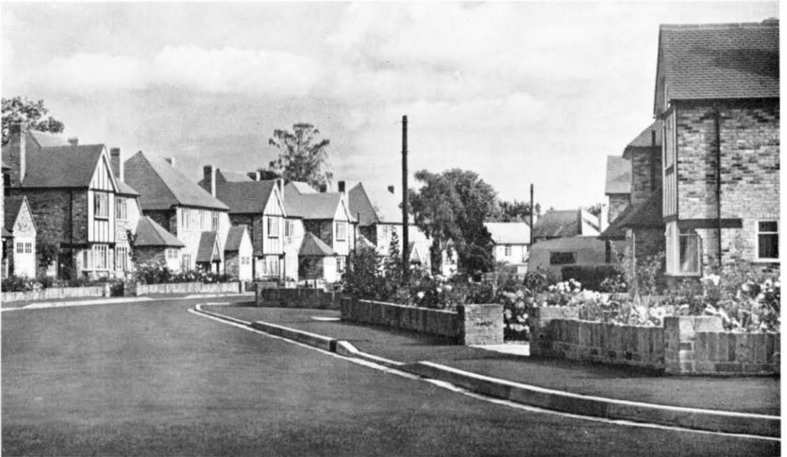
Modern overhead construction on a housing estate showing a medium pole and lightweight dropwire.
