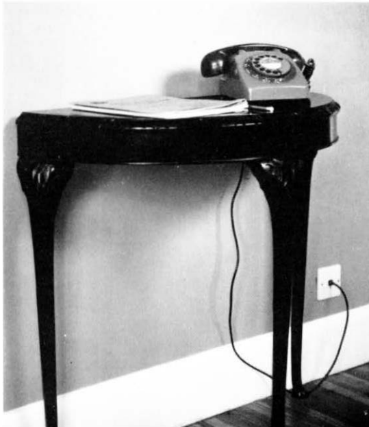
A new idea, tried out on some estates, is to provide a flush-fitting connection box in the wall so that a telephone can be connected without disturbing the house fabric.
