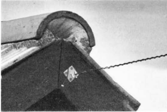
A modern external house termination which is much neater, smaller, easier to fit and less liable to damage than those previously used.
