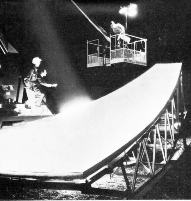
Left: Checking the accuracy of a petal by floodlight. The light reveals any irregularities in the reflector surface. Below: A view of the new aerial at Goonhilly seen from the earth station's control tower.
