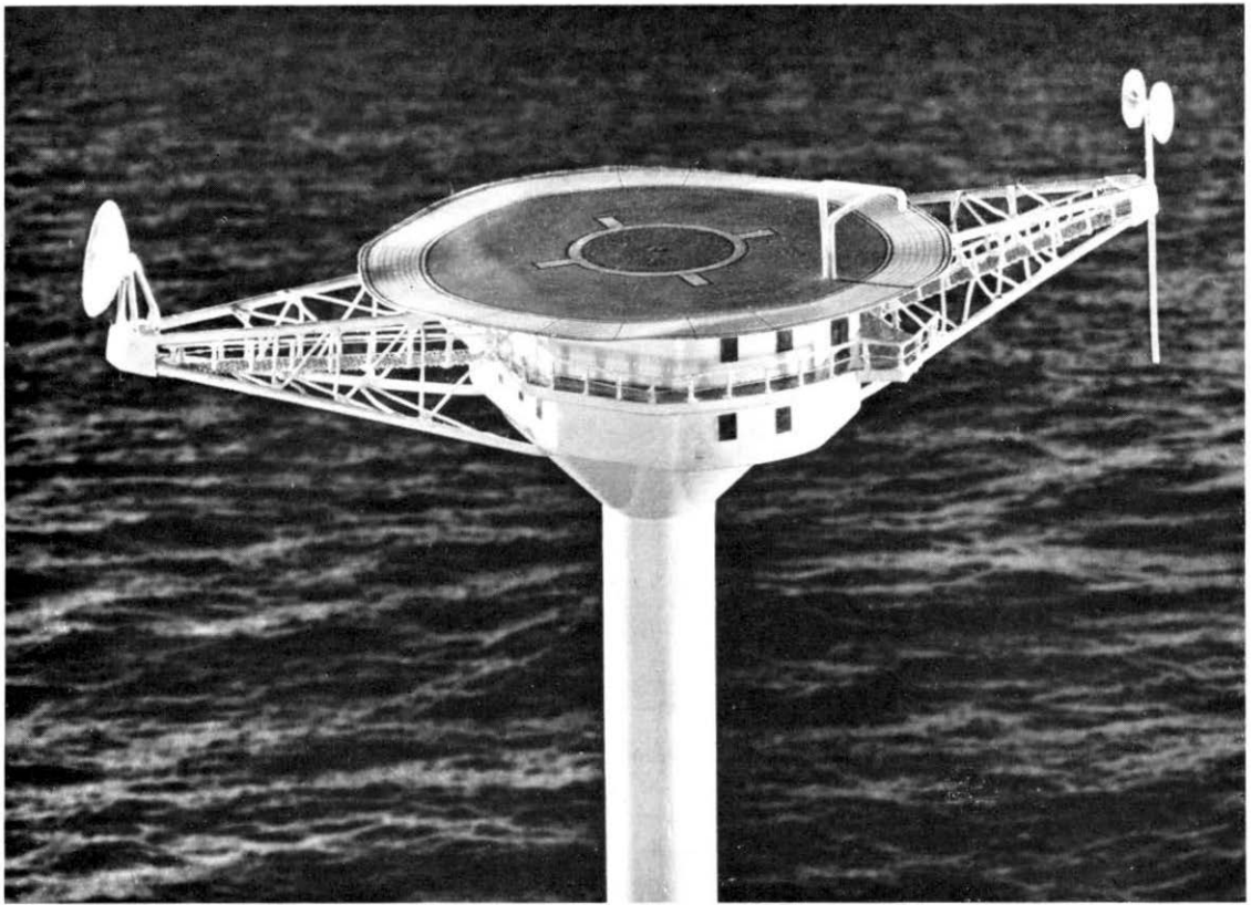
A scale model of one of the floating radio stations showing the aerials and, in the centre, a helicopter landing platform. The station would be about 400 feet long, most of it submerged
