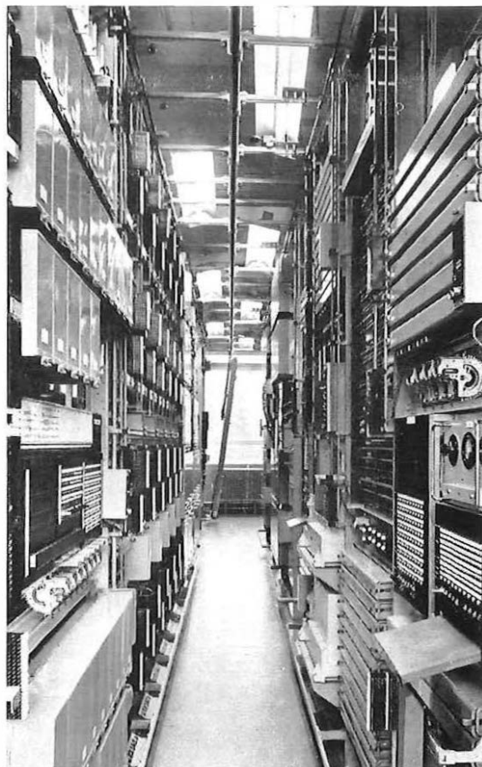
Part of one of the trunk units at Tunbridge Wells showing (left) M/U routiner registers and (right) register routiner pulse machines.
