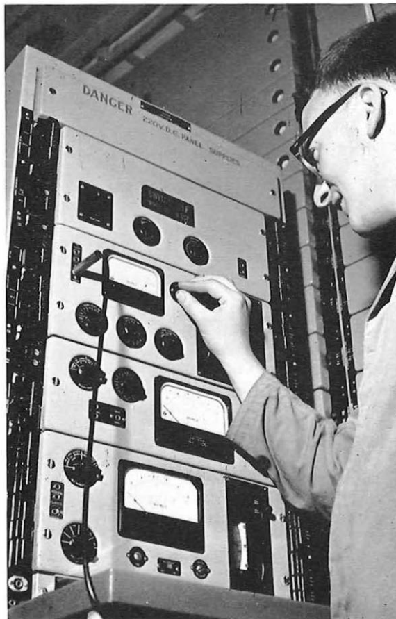
Measuring the high frequency response of a supergroup link (it can carry 30 simultaneous circuits) at the Reading centre.
