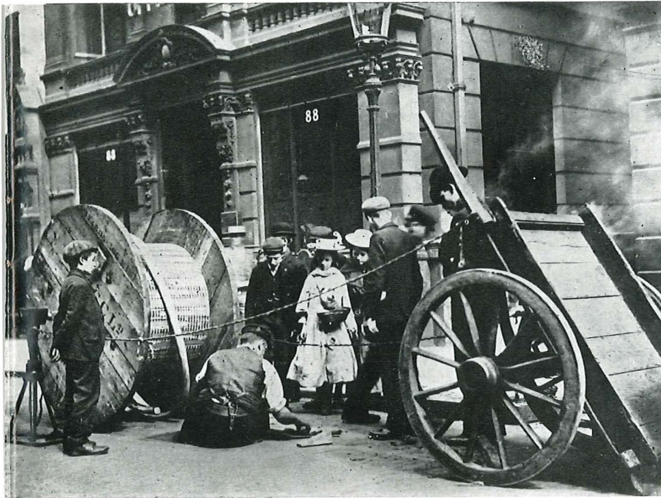
Under the fascinated gaze of a group of young spectators a cable-laying team of 1895 puts in new cables at Colmore Row outside the Central Exchange. Picture: Courtesy Birmingham Reference Library.
