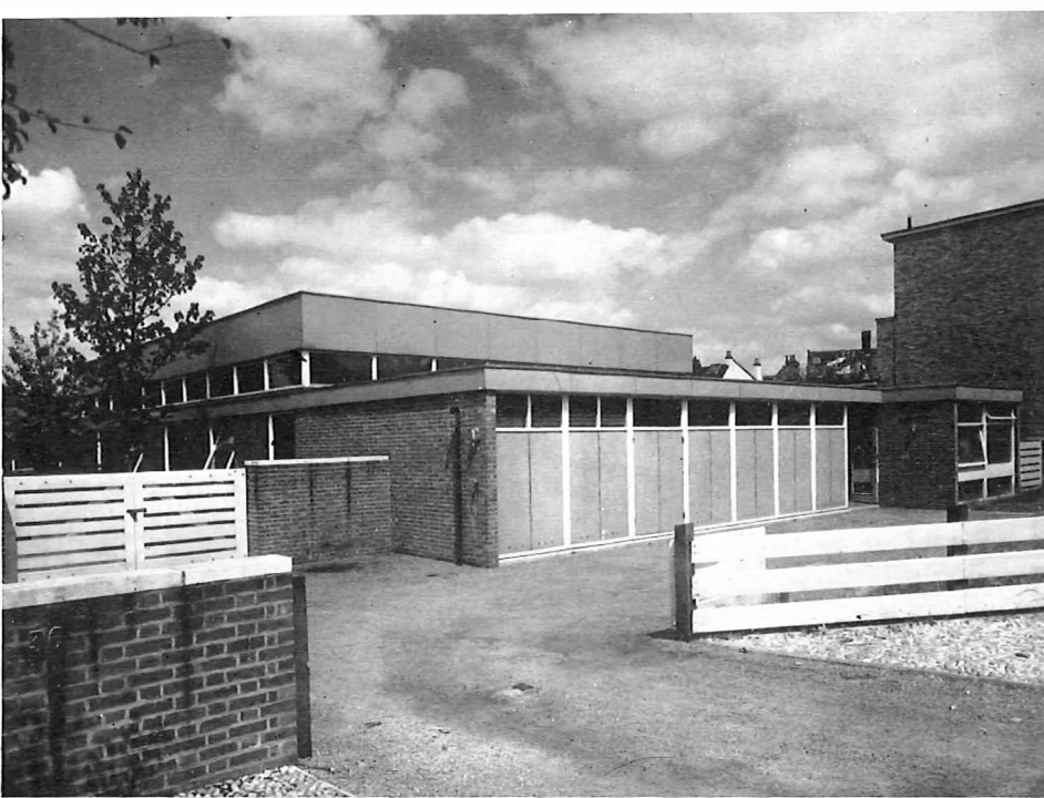
Left: The new K-type exchange at Beaconsfield, one of the first of the new range to be completed.
