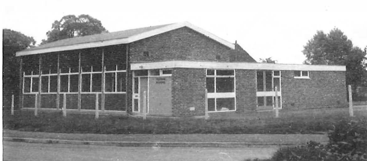
Left: A typical H-type telephone exchange building at Chestfield in Home Counties Region. The H-type is about the size of a normal bungalow.
