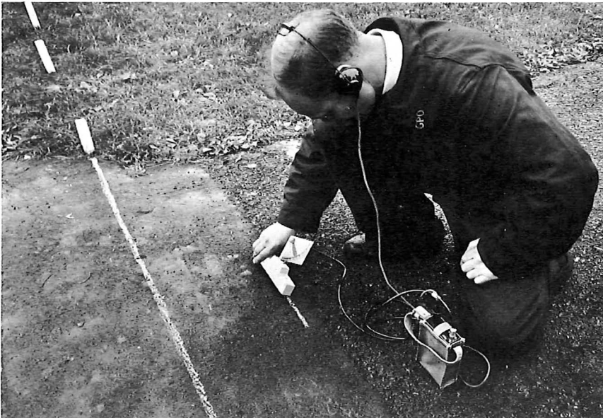
Measuring the depth at which a cable track is buried. The search coil is tilted to discover the angle of minimum tone and the indicator shows the exact depth.
