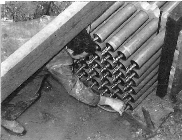
Above: A workman places spacers over the PVC ducts so that they can later be built into a nest. Below: Pressurising the ducts of a 36-way formation nest before the concreting operation is carried out.
