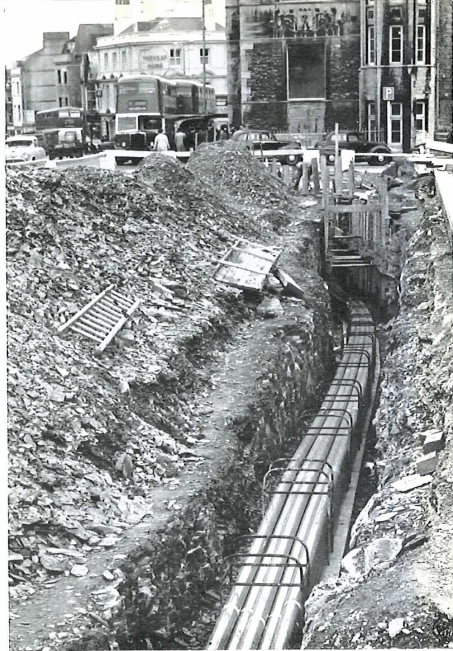
During recent trials with PVC duct, an 18-way, closed formation track was laid in Plymouth. Above: The PVC track before the walls and roof were concreted. Below: Vibrating concrete round the PVC pipes.
