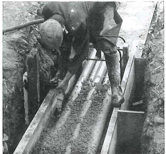
During recent trials with PVC duct, an 18-way, closed formation track was laid in Plymouth. Above: The PVC track before the walls and roof were concreted. Below: Vibrating concrete round the PVC pipes.
