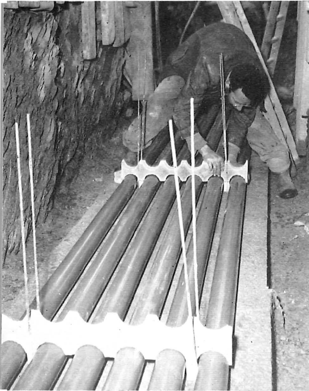
Above: A workman places spacers over the PVC ducts so that they can later be built into a nest. Below: Pressurising the ducts of a 36-way formation nest before the concreting operation is carried out.
