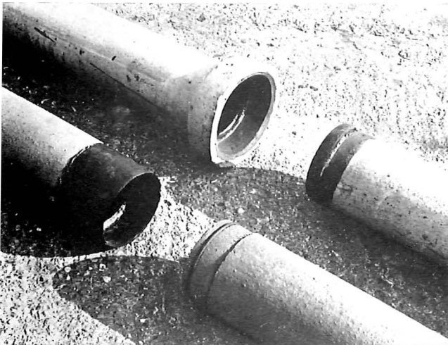
The new duct joint (foreground) showing the sealing ring and plastic socket. Behind it, the standard Stanford composition joint of the present Duct No. 5.
