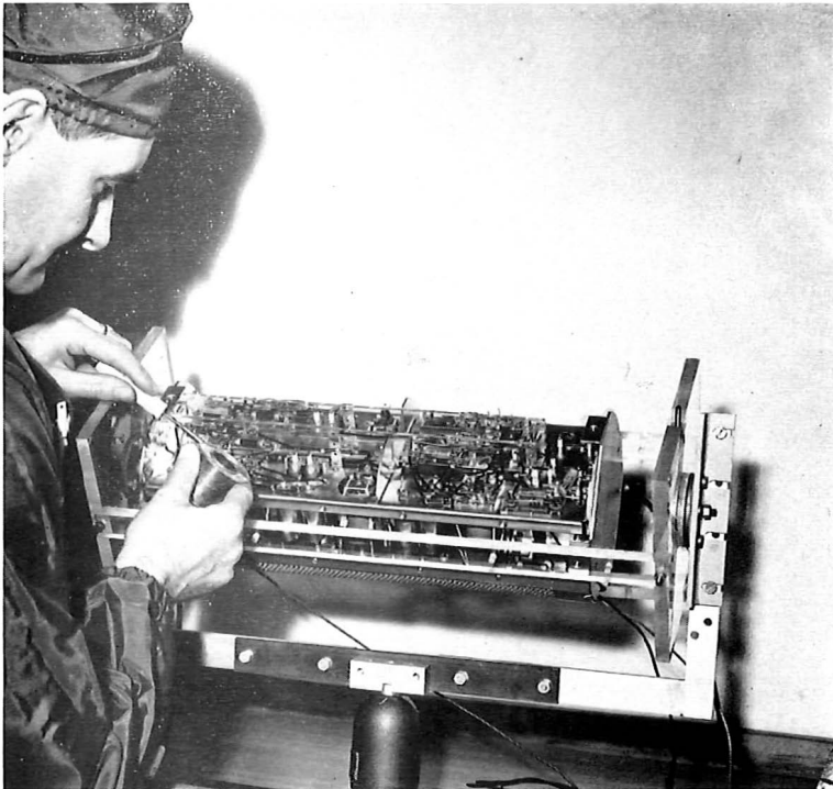
A dismantled amplifier, mounted in a special jig to reduce the risk of damage, undergoes repair. Note nylon hat and overalls.
