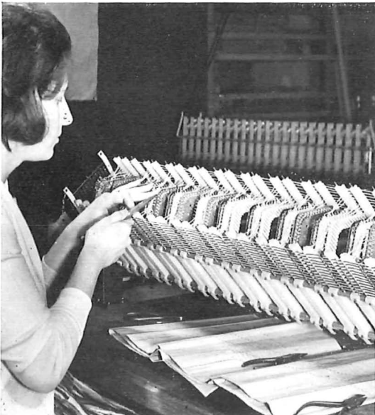
A view of one of the units of a time-division electronic exchange being wired.
