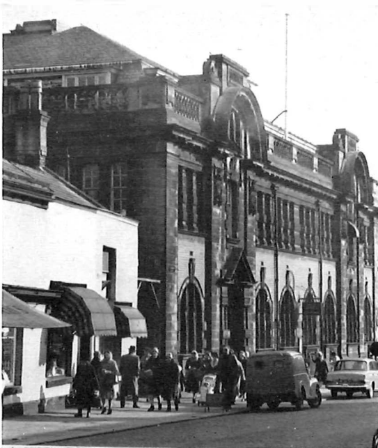
◀ The Blackburn Head Post Office which houses the 48-year-old automatic exchange and plant.
