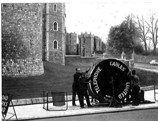
T.C.L. moisture barrier cable at Windsor Castle
