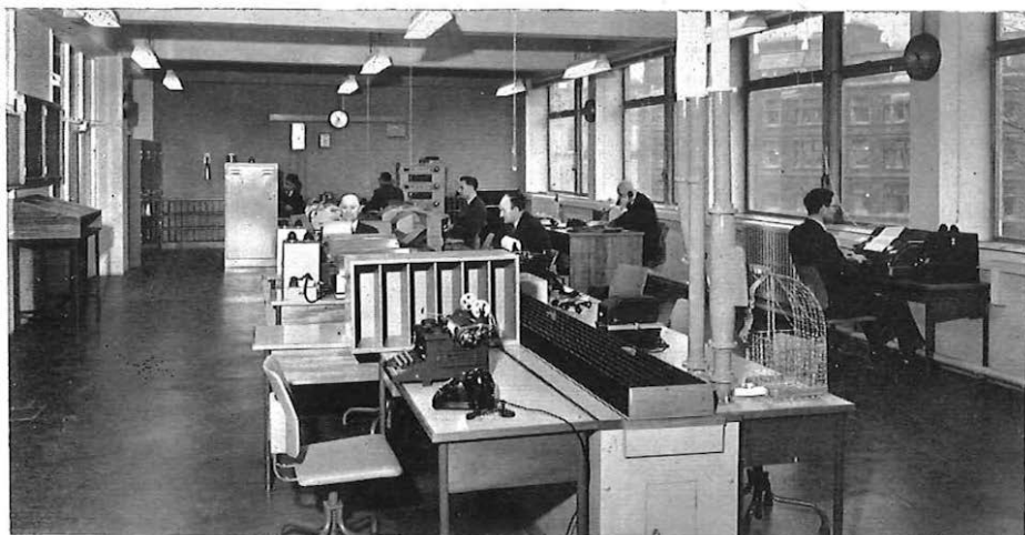
Another view of the new overseas telegraph area office at Broadway, SW1, showing three-tier teleprinter stacks for Gentex traffic in the background.
