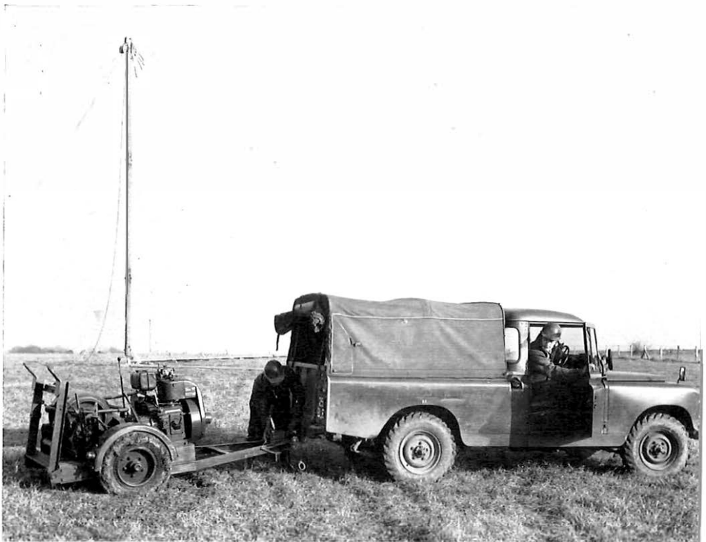
Above: A 150-ft high steel lattice mast at Leaffield is hauled into place by the winch. Below: Task completed, the winch is attached to its Land-Rover and driven away.
