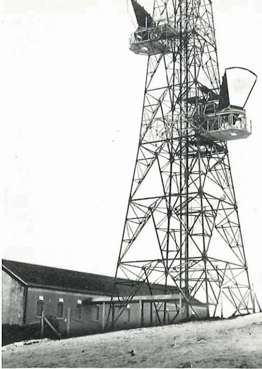
A tower at Riddings Hill Radio Station showing the new horn reflectors which enable aeri-als to be shared by several frequency bands.
