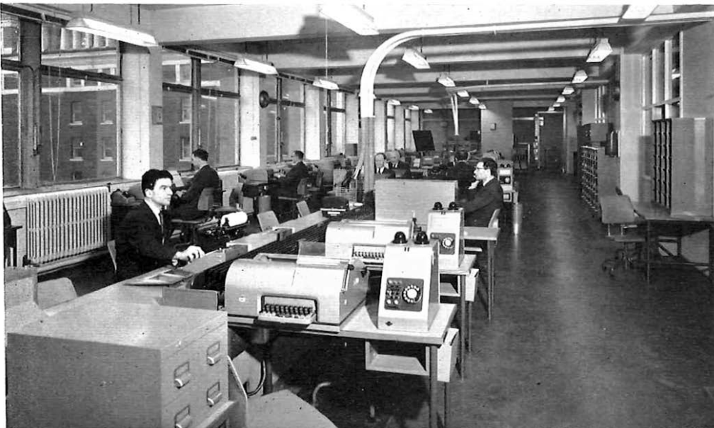
A view of the delivery suite at the new overseas telegraph area office at Broadway, London, SW1. A multi-track conveyor belt system routes messages from overseas to the various delivery positions (telex, in foreground), phonogram and via pneumatic tubes for delivery to postmen.
