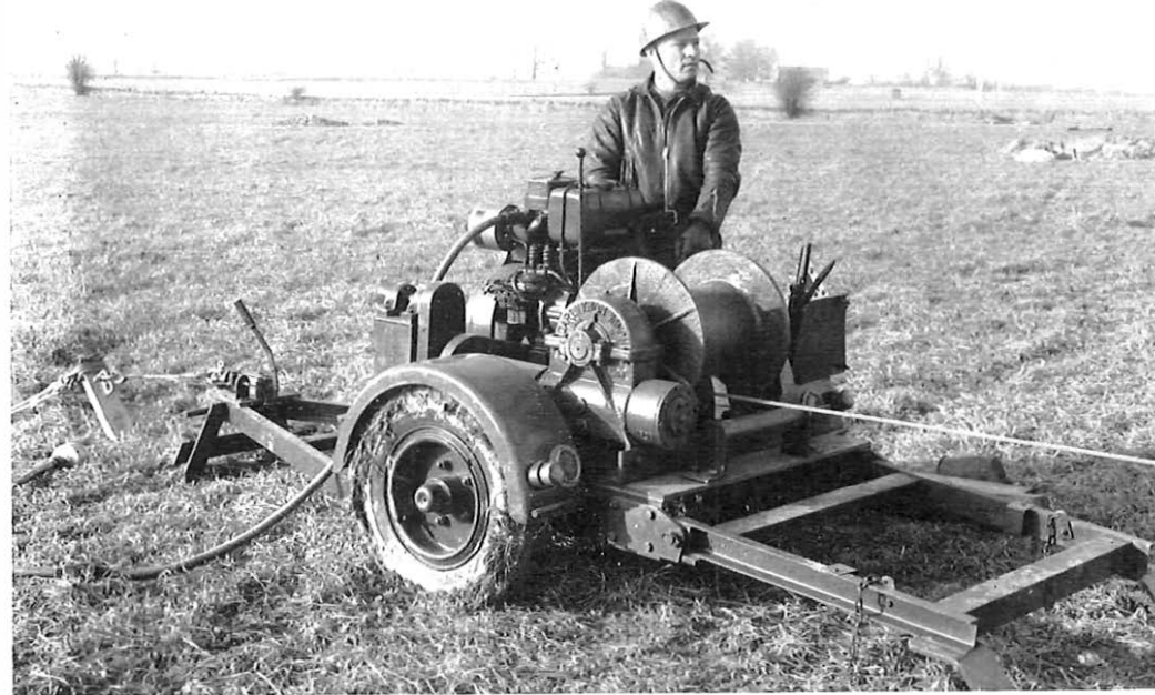
A close-up of one of the new winches as it is made ready to erect a radio mast at Leaffield. The winch drum can carry up to 1,100 feet of steelwire rope.
