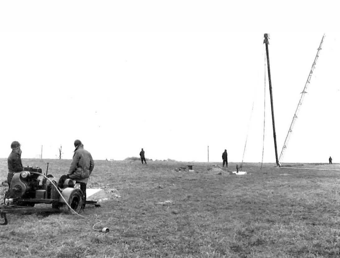
Above: A 150-ft high steel lattice mast at Leaffield is hauled into place by the winch. Below: Task completed, the winch is attached to its Land-Rover and driven away.
