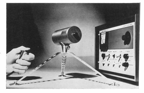
The Hughes I Ib laser undergoing a test. It emits an almost parallel beam of light brighter than the sun.—Courtesy, Hughes International (UK) Ltd.
