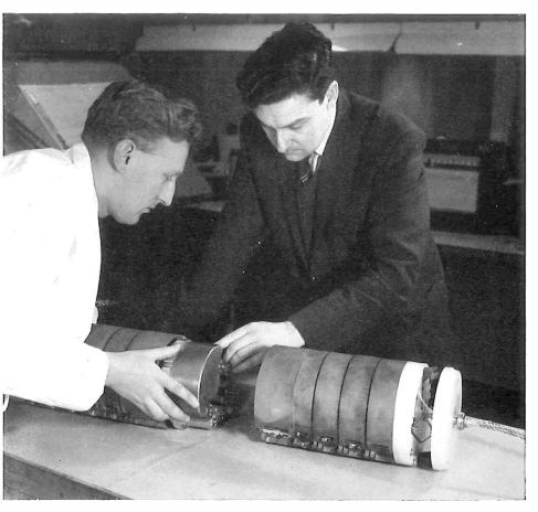
Assembling one of the newly-developed transistor submerged repeaters which will be used in one of the Anglo-Belgian cables to increase its capacity from 216 to 420 circuits.—Courtesy: Submarine Cables Ltd.
