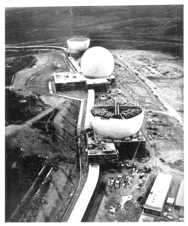
An aerial view of the three giant radomes, the centre one completed, at Fylingdales. The radomes protect the tracking radar aerials and each is made up of 1,646 panels.
