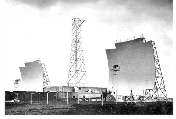
Two radio reflectors (left and right) which are part of the communications system.
