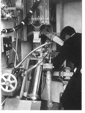
An engineer inspects the maser and its associated apparatus and waveguides at the Post Office Satellite Systems Ground Station at Goonhilly.
