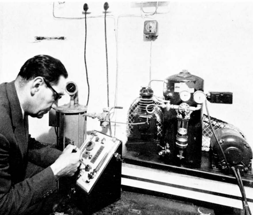
An engineer checks the dryness of the air in the cable at the Deal end by extracting a small part of the air and measuring the dew point. On the right of the picture is the compressor equipment.
