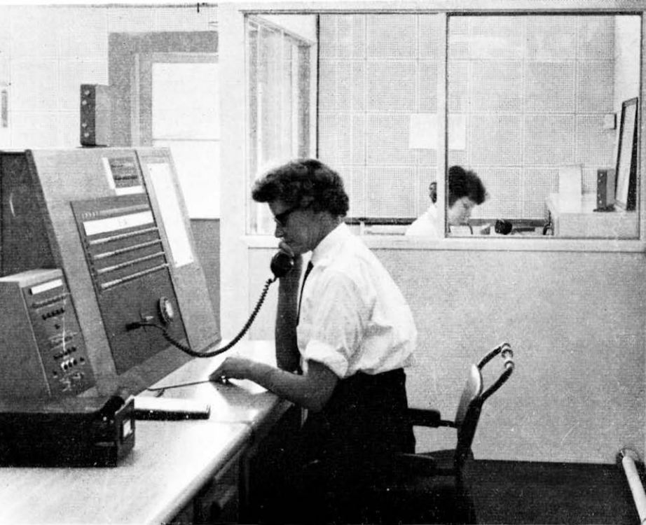
The new Voice Frequency Remote Control equipment (extreme left) on field trials at the Control Room of Kent County Fire Brigade HQ in Maidstone. Alongside the equipment is one of the cordless PMBXs which have been developed for the Fire Service by the Post Office.
