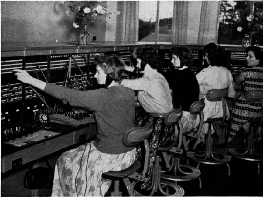
Operators at the Weybridge Exchange connecting trunk calls.
