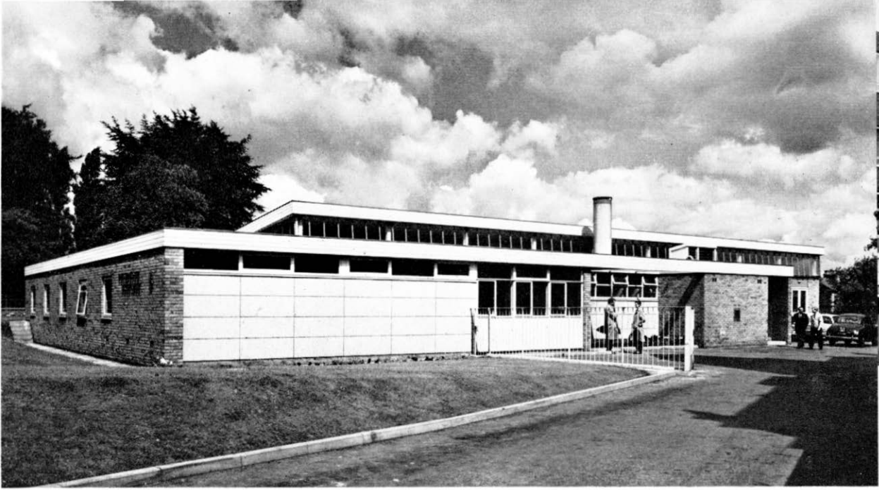
The Altrincham automatic telephone exchange—a fine example of the new approach. It was built at about half the cost and in much less time than any other similar exchange.
