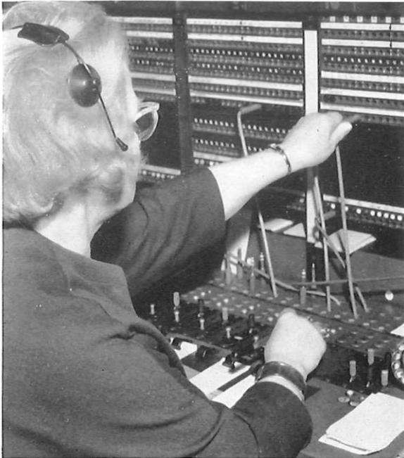
The London Continental Control Centre at Wood Street is equipped with a low-type multiple.
