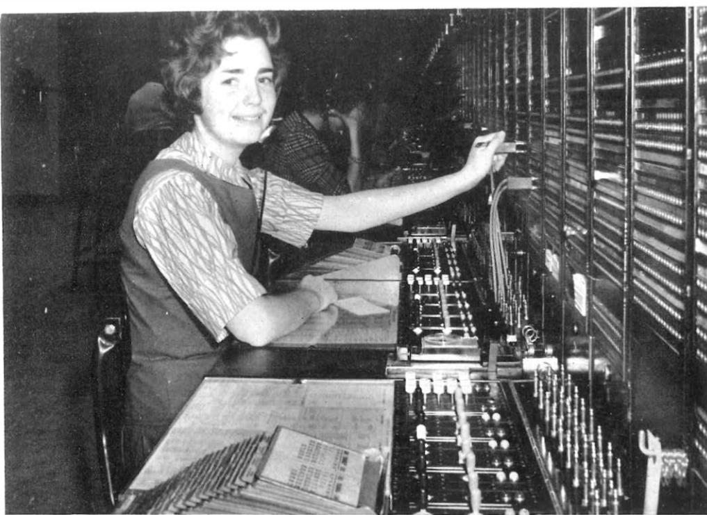
Right: An operator at the International Exchange in London dialling a New York White Plains operator. Note the double-ended cables connecting the United States to the United Kingdom. Note, too, the
