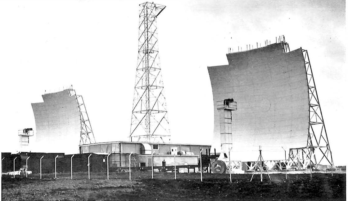
Two radio reflectors (left and right) which are part of the communications system.
