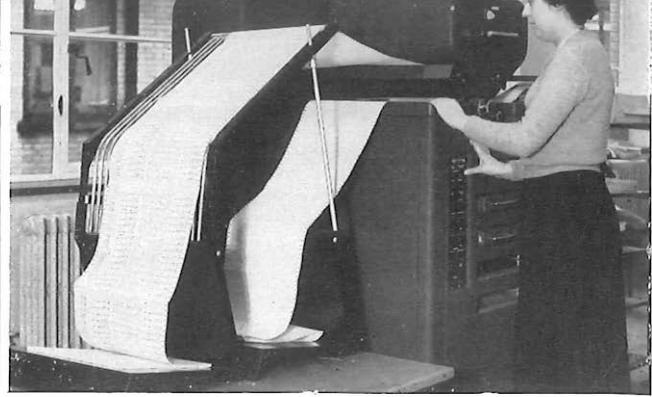
Two pictures of the Post Office's own LEAPS computer system. Left: An operator prepares data in punched tape form for input to the computer. Right: Payroll documents for issue to local pay units being printed by one of the two high-speed Samastronic printers. The printhead shown here is driven electrically from magnetic film on which payroll details have been recorded by the computer.
