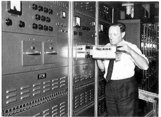
Above: Mr. A. Wilkinson, GPO Technical Officer, adjusts an amplifier in one of the power supply units.
