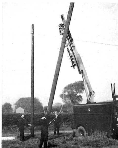
Perched in a bucket at the end of the derrick an operator demonstrates how he can raise himself aloft. The derrick can also be used for erecting new poles and lifting out old ones, handling stores and steering the pole hole borer.
