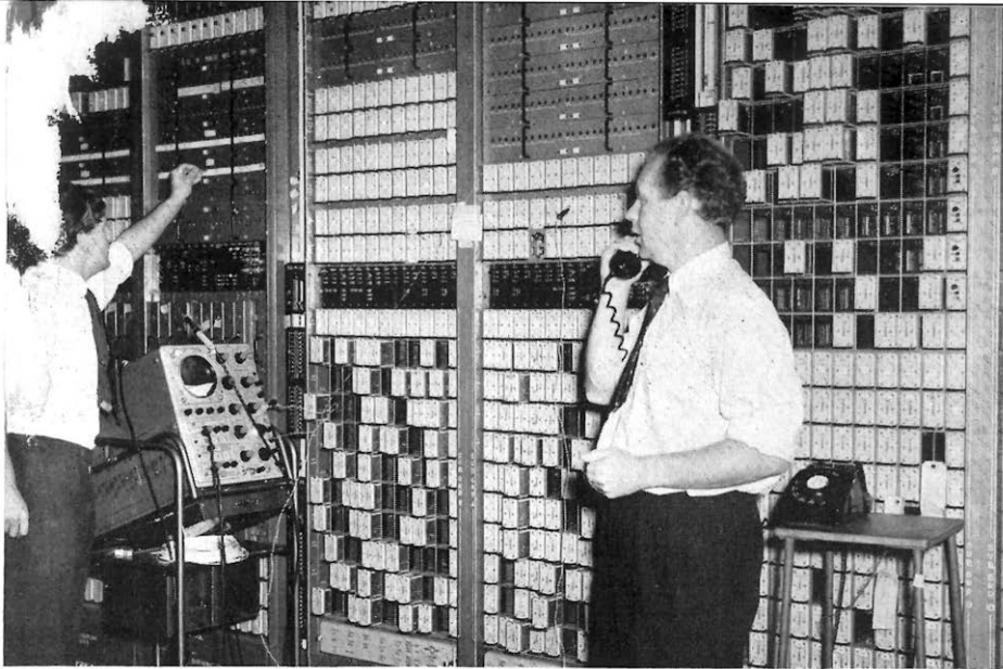
Mr. E. Peddle (left), GEC, and Mr. Bruce Looms, AE at Dollis Hill, at the speech multiplex rack. Each call going through this rack is cut into one-hundredths. Mr. Peddle is plugging in an oscilloscope to monitor pulses as they pass through the equipment.
