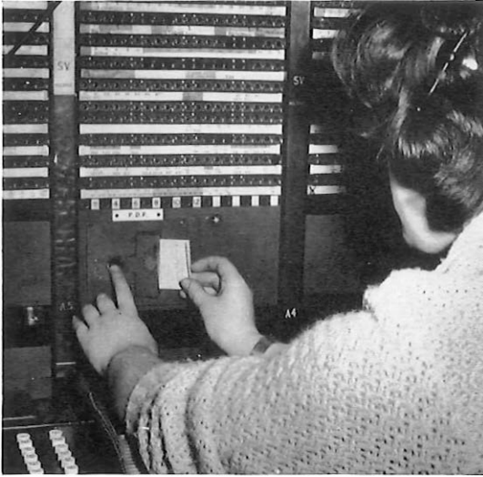
Sending a ticket by pneumatic tube to the Pneumatic Distribution Position at Continental Exchange.
