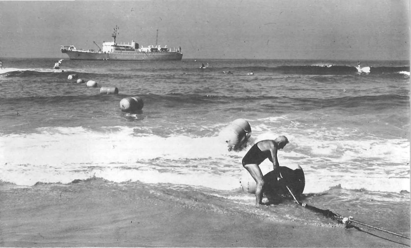
Beach-inspector A. Laidlaw, who swam out from Bondi Beach to bring ashore the cable carrier line, attaches it to the armoured cable.
