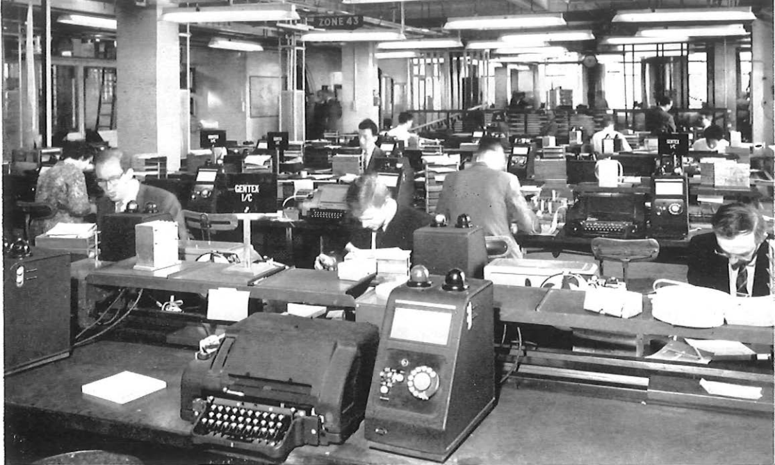
Operators at work in the Incoming Gentex Section. In this office all incoming messages are received on tape machines and then gummed down on forms for delivery to the recipients in the normal manner.
