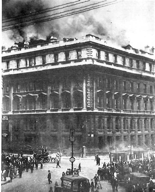
The CTO blazes after being hit by a German bomb in 1917. But the damage was negligible compared with that sustained in World War Two. This picture was taken from Cheapside.
