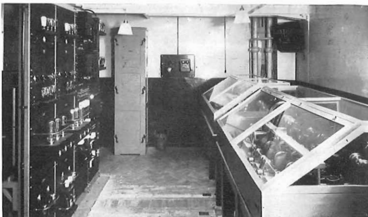
The TIM speaking clock installed at the Holborn Exchange in 1936 and which still shows no signs of wearing out.
