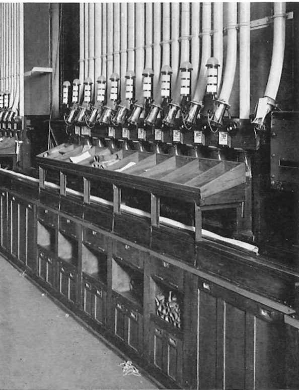
Pneumatic tube terminals at the CTO main circulation point in 1935. The three lamps for each tube showed whether it was in use for an outgoing or incoming call or disengaged.
