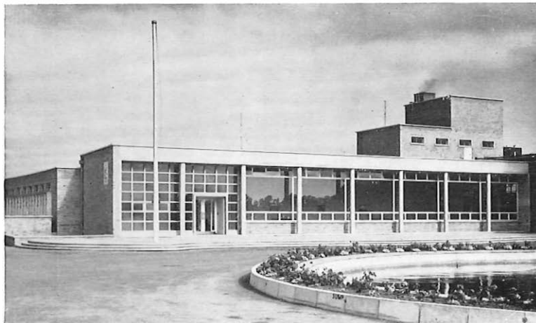
Right (above): Preparing a telegram in Electra House in 1960 for radio transmission to Karachi. Below: One of the newer Rugby Radio station buildings.
