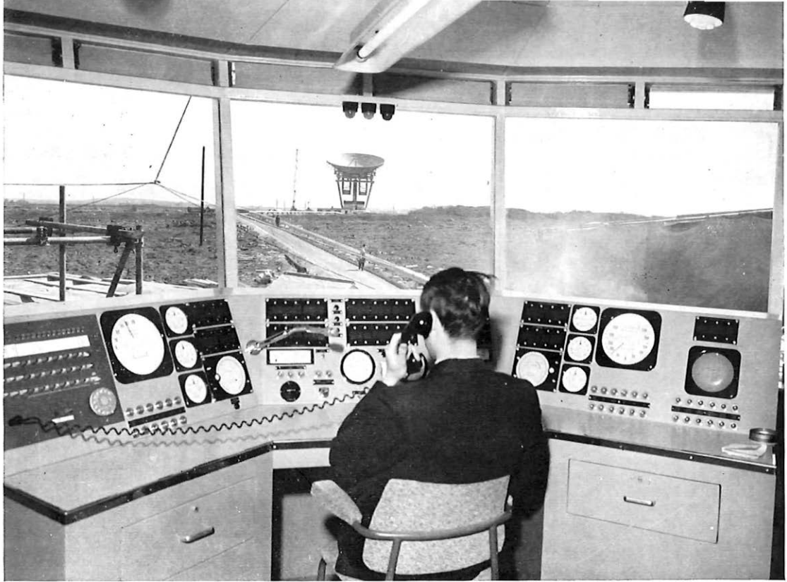
The aerial steering room in the Control Tower at Goonhilly. From here an engineer keeps watch over the station, corrects faults indicated by the instruments in front of him and, if necessary, steers the giant aerial.
