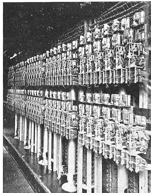
BELOW: The connector side of a line switchboard of the same period, showing five units with 12 connectors for each unit.
