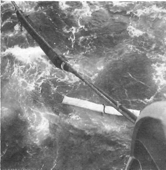
Repeater leaves stern sheave and parachute bag falls clear
