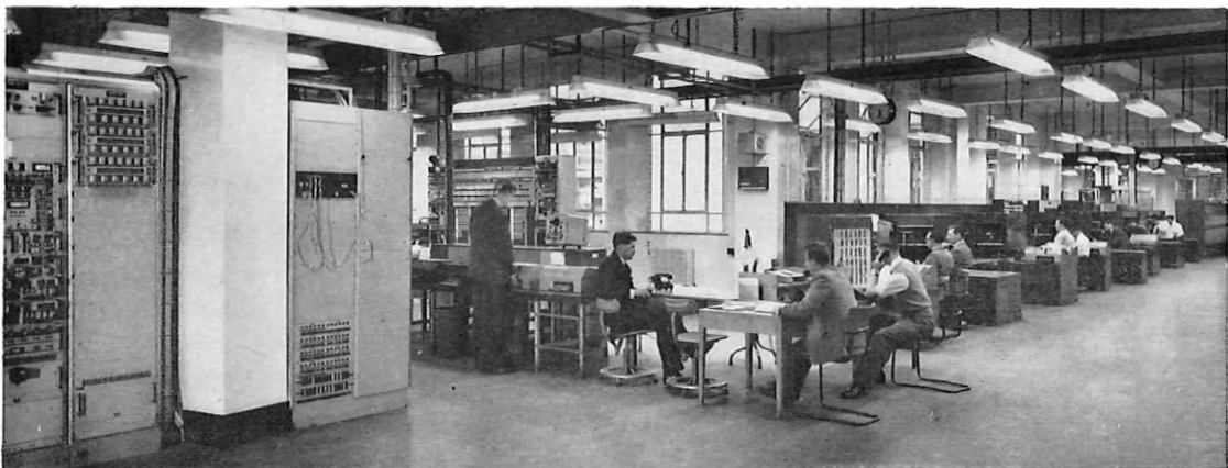
Fig. 1: The Control Room in Electra House
