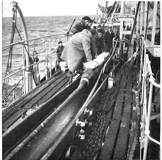
Repeater approaches stern sheave
