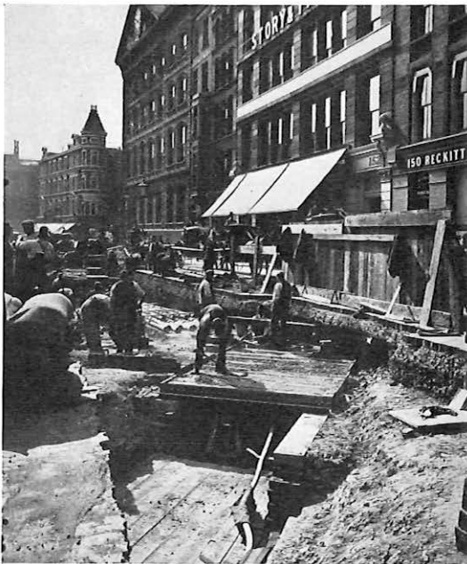
1901: Laying underground cable in London
