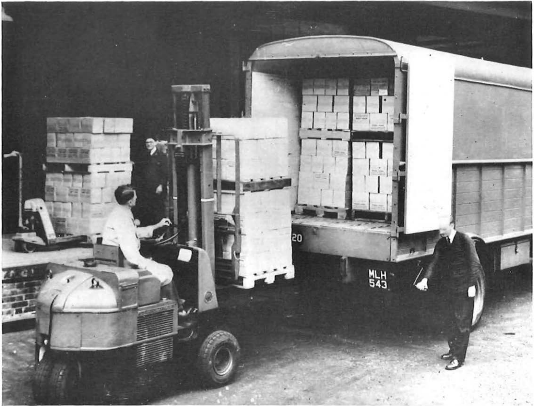
Fig. 3 : Moving-floor van. Loading and unloading area always presented to tail-board
