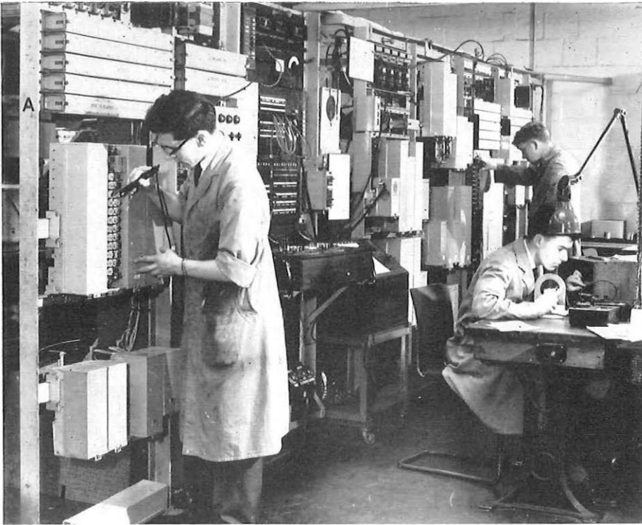
Equipment for the Continental semi-automatic system undergoing tests in the Laboratory
