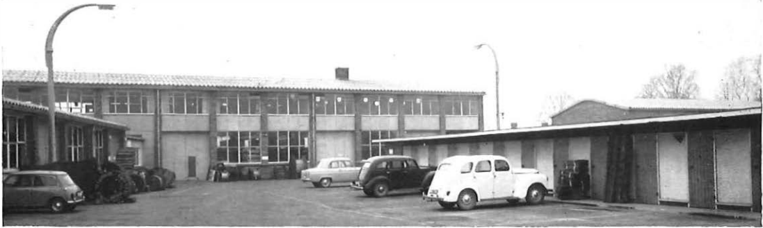
Fig. 2: Two-storey building with offices and welfare rooms above the covered storage area
