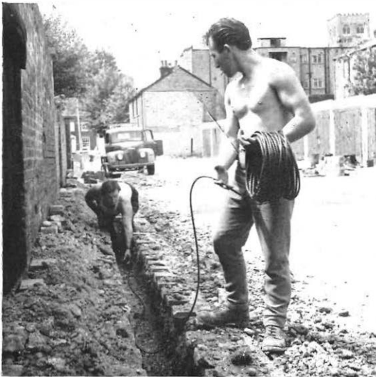
Fig. 3: Contractor's men laying polythene cable in footway
