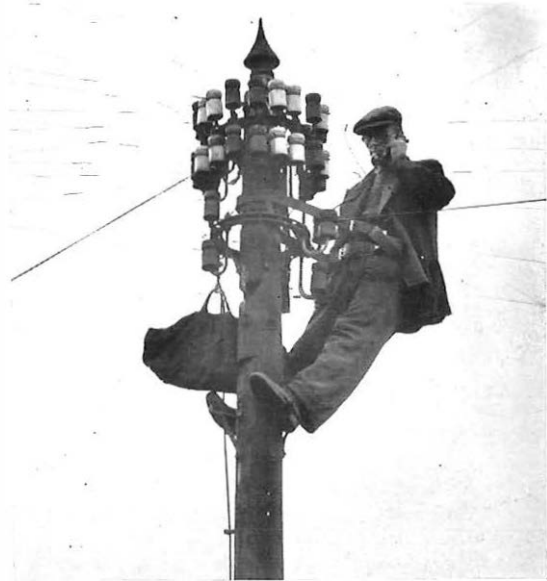
Fig. 5: Technician working on pole-head of ring type distribution pole
